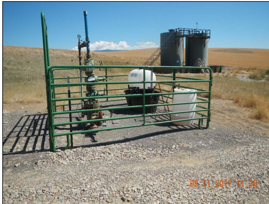
Photo 1. Chemical tote without secondary containment.
