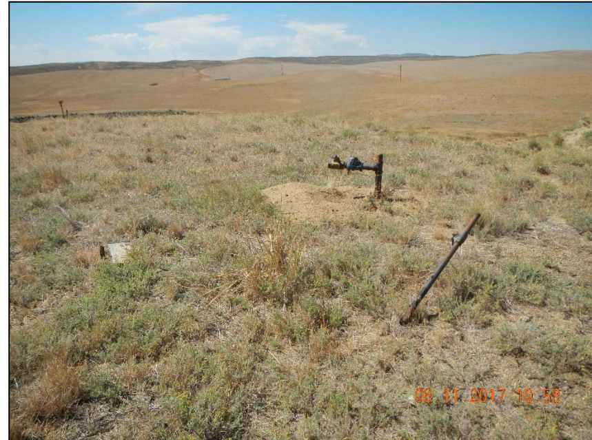
Photo 3. 2 – 1" steel risers and 1 – 2" steel riser.
