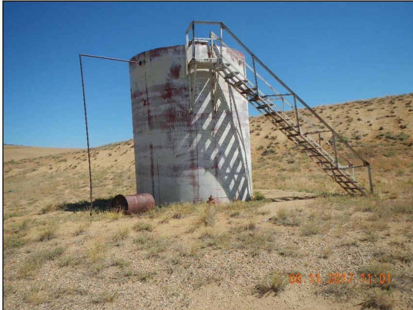
Photo 4. Tank with no label and no berm. Container with no secondary containment next to tank.
