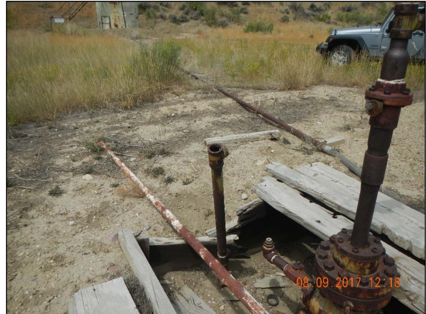
Photo 2. 2" riser at wellhead.
