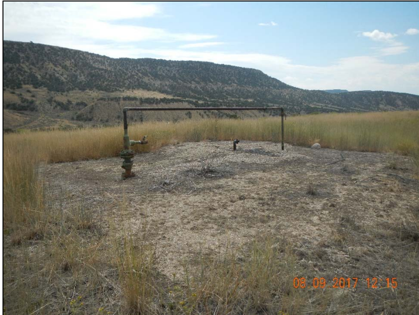
Photo 1. 3 – 2" steel risers on location.
