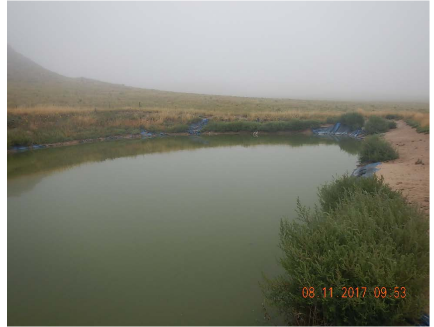
Photo 3: Pit liner sagging
