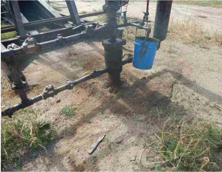
Photo from prior inspection for comparison
