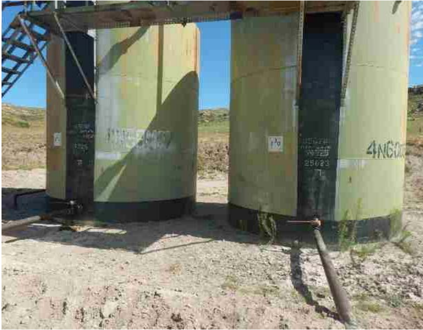
Photo from prior inspection for comparison
