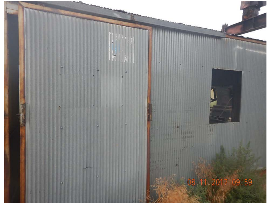
Photo 4: Prior operator signage removed
