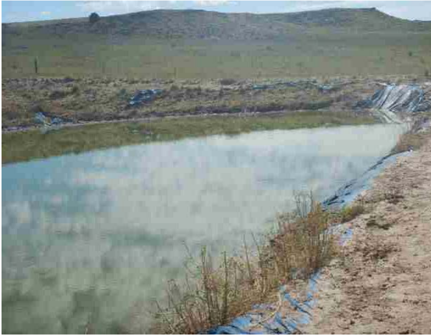
Photo from prior inspection for comparison
