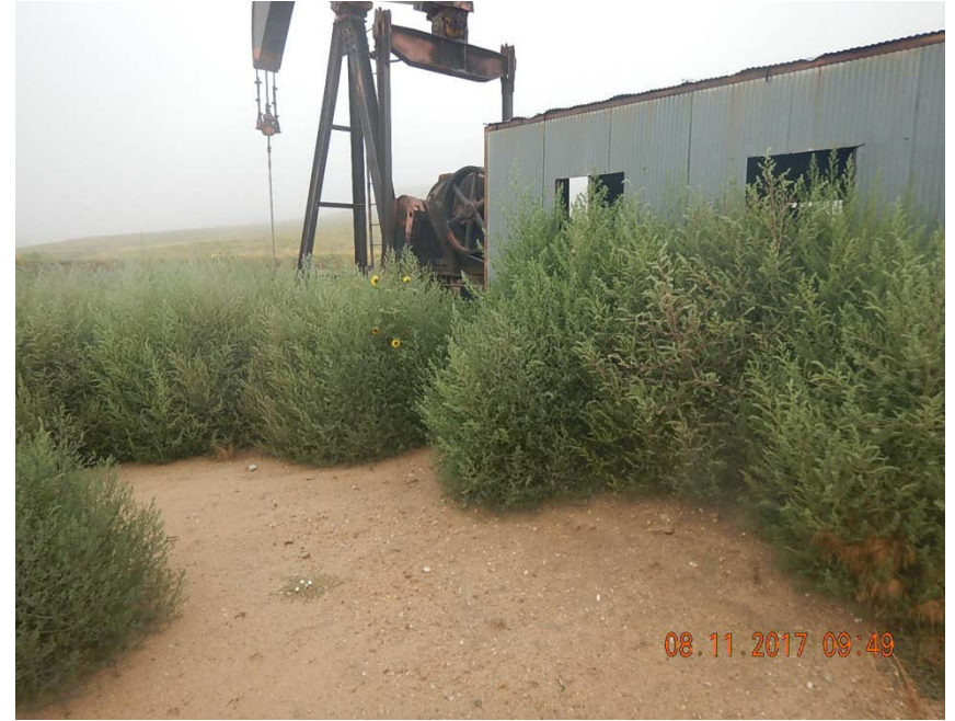
Photo 1: Weeds around wellhead and engine. Cannot determine soil status around wellhead.
