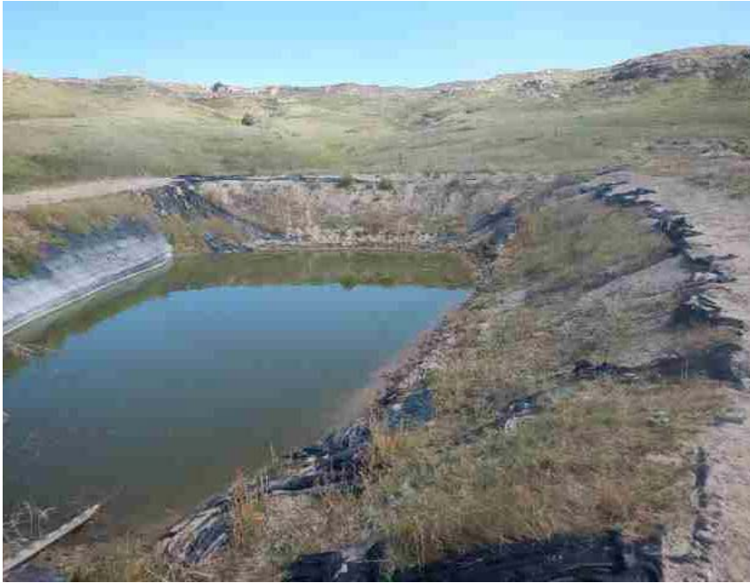
Photo from prior inspection for comparison
