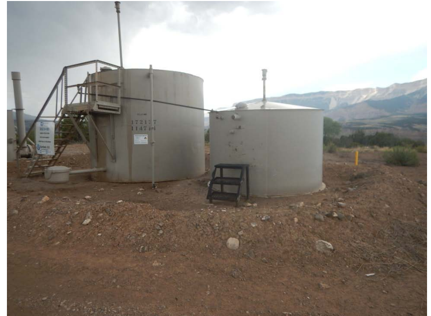
Small tank with no labels or placards noted in previous inspection as Corrective actions needed
