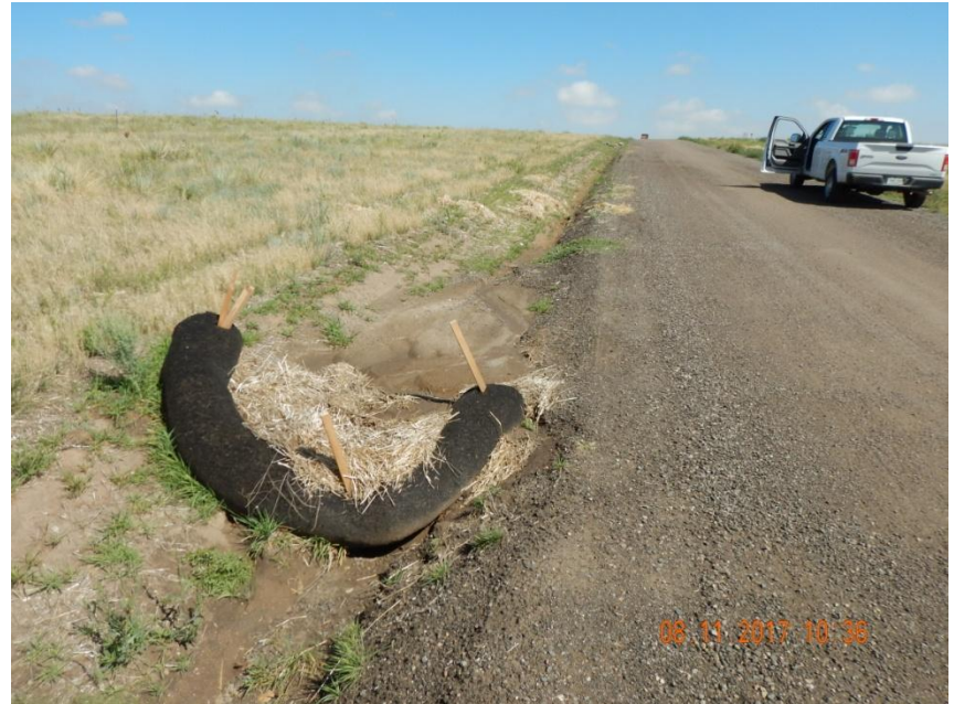
Photo 6. Photo taken north of the culvert crossing on the west-side of the main access road, facing North. BMPs in need of maintenance as the wattles are full of sediment.
