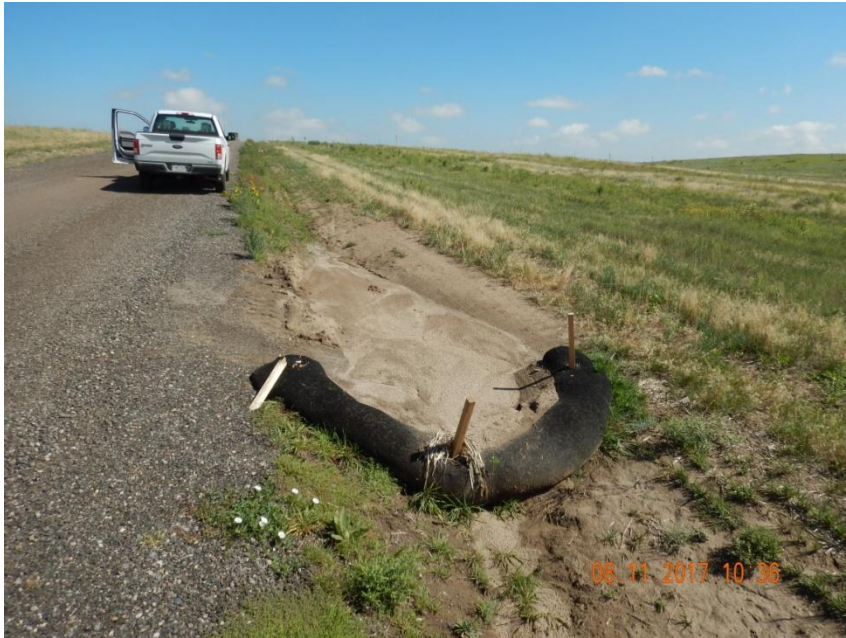
Photo 5. Photo taken north of the culvert crossing on the east-side of the main access road, facing North. BMPs in need of maintenance as the wattles are full of sediment.
