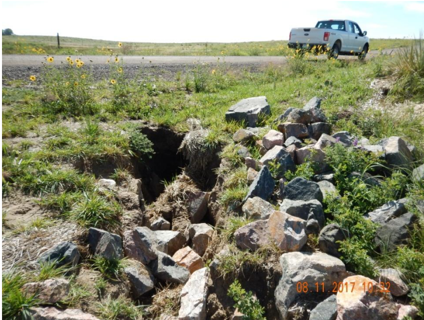
Photo 3. Photo taken along the west-side of the culvert crossing, facing Southeast. Erosion (head cut) forming along the west-side of the culvert area. Need to stabilize and prevent erosion from occurring.
