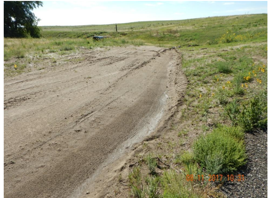
Photo 2. Photo taken from the previous photo location, facing South. Sediment deposition observed from stormwater erosion along the access road. Need to control and stabilize this area of sediment deposition so it does not erode into the intermittent stream.
