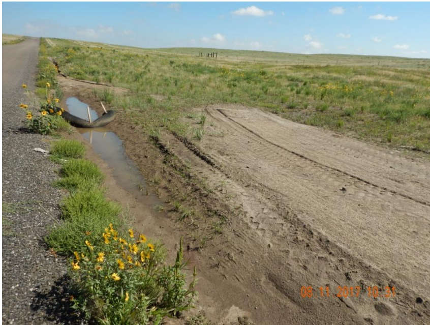
Photo 1. Photo taken just north of the culvert crossing, facing North. Sediment deposition observed from stormwater erosion along the access road. BMPs along the access road in need of maintenance.
