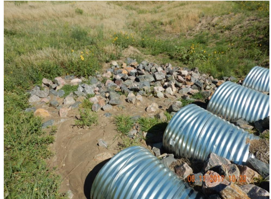
Photo 4. Photo taken along the west-side of the culvert crossing, facing West. Sediment deposition occurring along the outlet area. Maintenance required as this sediment could potentially discharge from the outlet area and contribute to sediment discharge into Box Elder Creek downstream.
