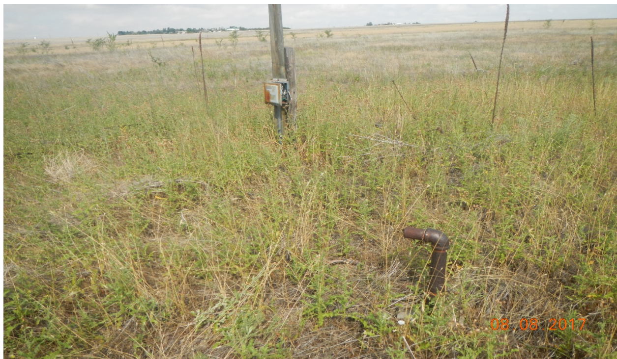
photo 2: There is a pipe riser and an electric utility that remains at the west side of the location. Lat/Long:39.78410,-104.36549.
