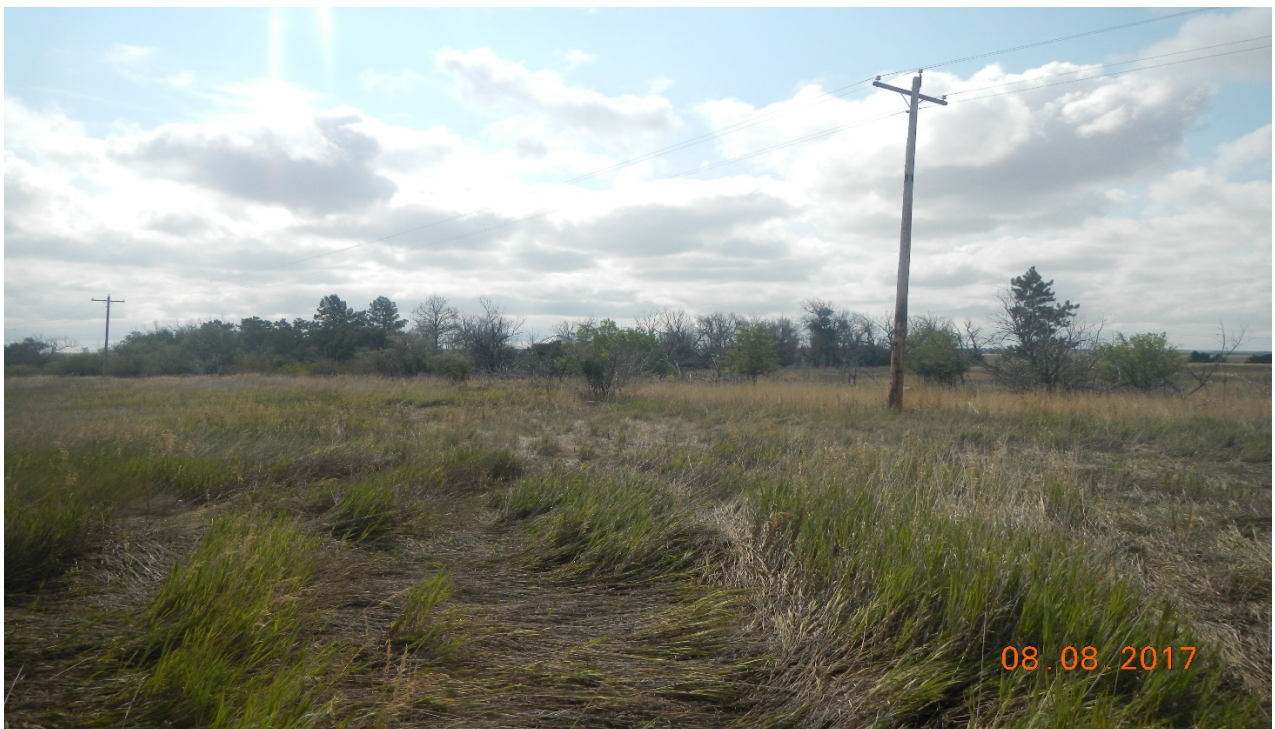
photo 4: The electric utility to the location appears to have been removed however, the main powerline remains.
