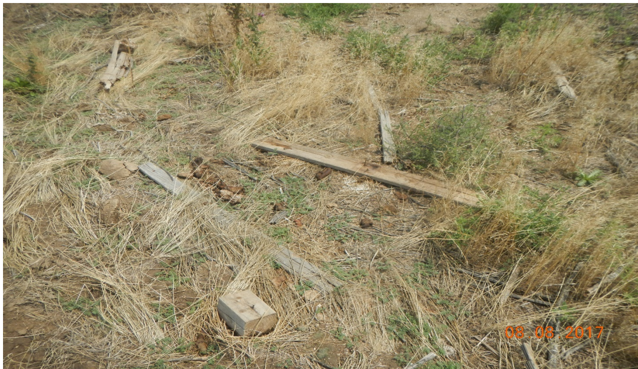
photo 3: There is wood boards and various debris that remains.
