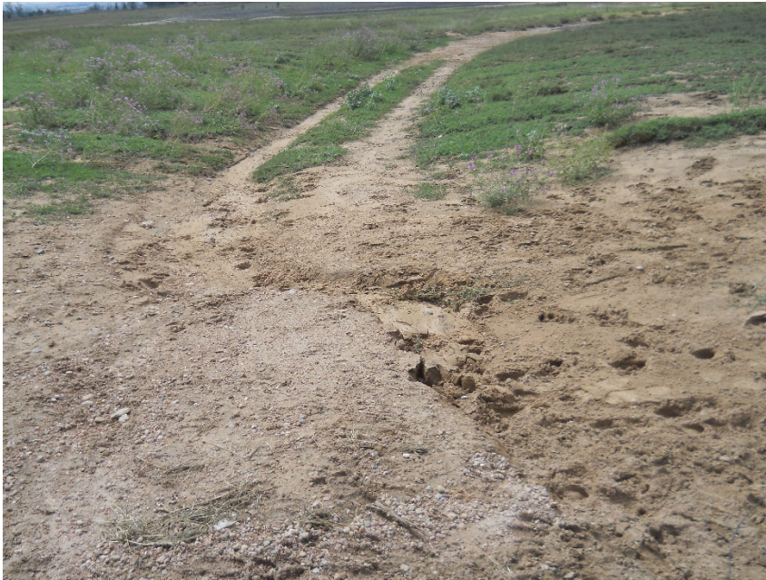
Battery entrance looking south. Lease road washing out, carrying sediment off.
