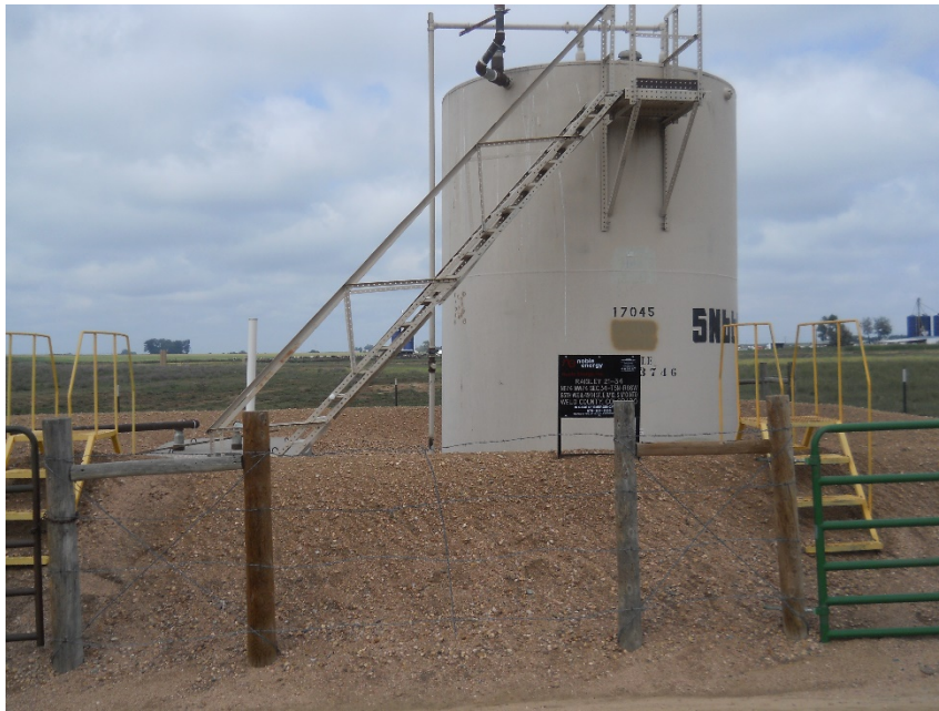
Tank battery looking north
