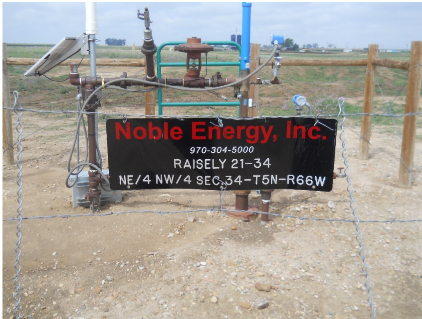
Wellhead sign looking west
