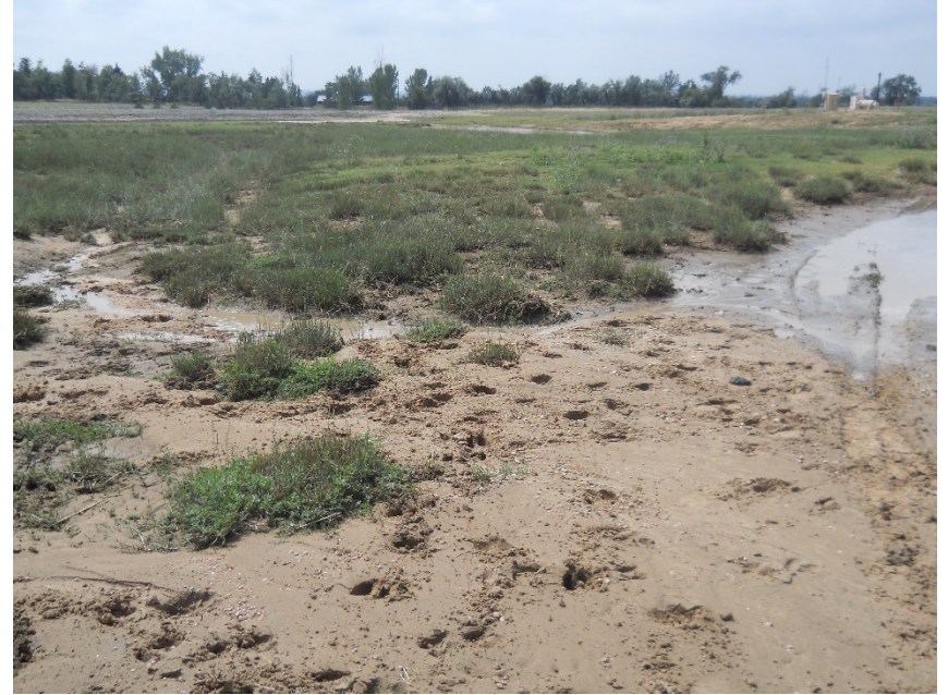
Lease road looking south before curve. Standing water actively draining through lease road to the east
