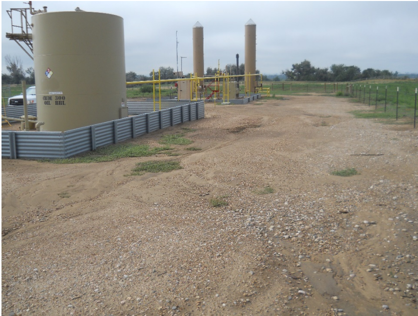
Northwest edge of location looking south. Location washing out from northwest edge around west side of production tank and discharging off of southeast edge of location
