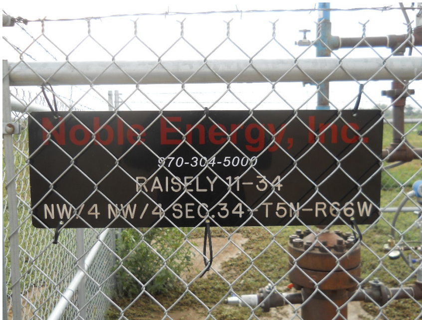
Wellhead sign looking east
