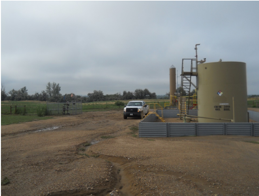
North edge of location looking south. Location washing out
