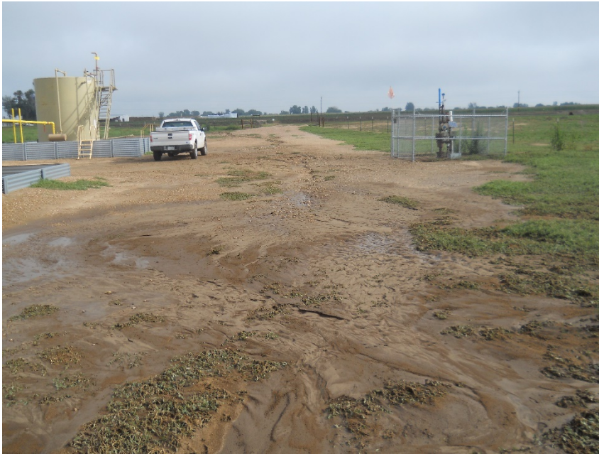
Southeast edge of location looking north. Location is washing out from the north edge and discharging off the south/southeast edge of location. Sediment carry off of location
