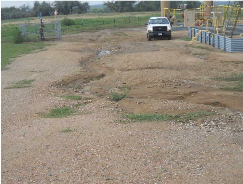
Location entrance looking south. Location washing out and discharging east at wellhead and south edge of location
