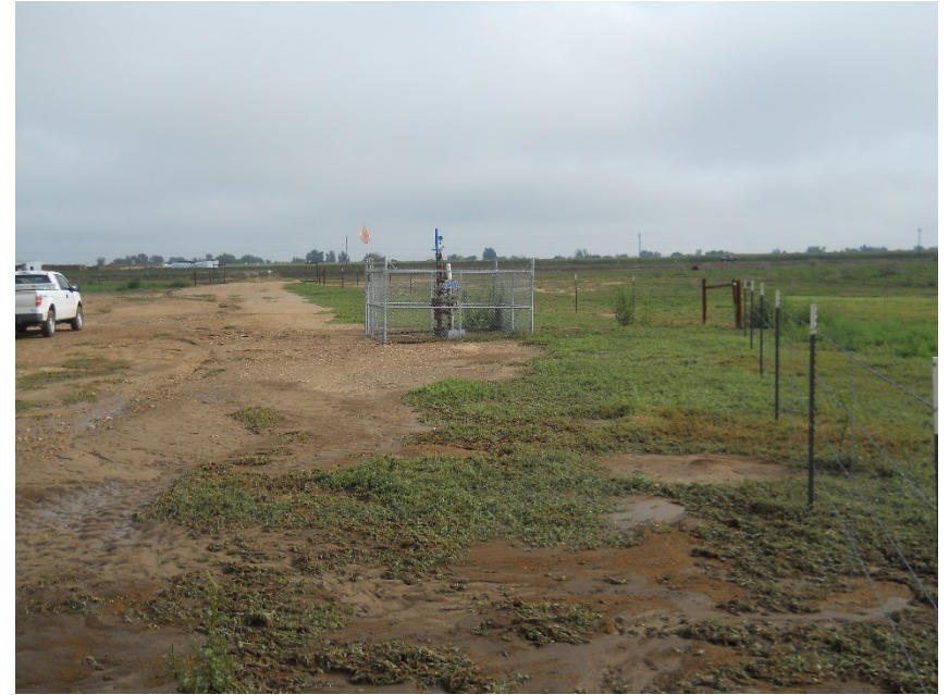
Southeast of location looking north. Weeds need to be controlled
