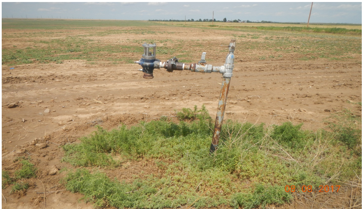
photo 2: The levers remain and no lock out/tag out has been applied.
