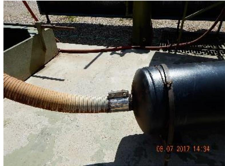
Photo 14: Flex pipe connection to in-line muffler.
