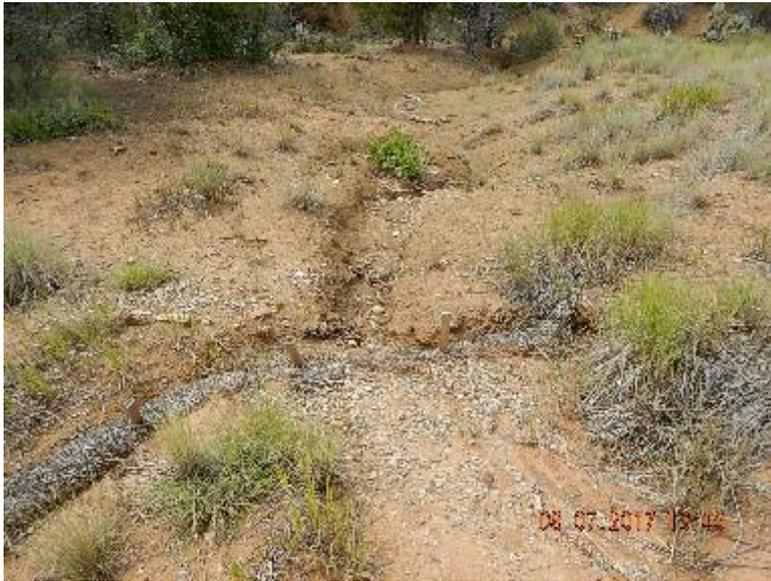
Photo 9: Full waddle and erosion channel.
