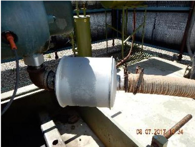
Photo 13: Muffler and connections at pump jack motor.
