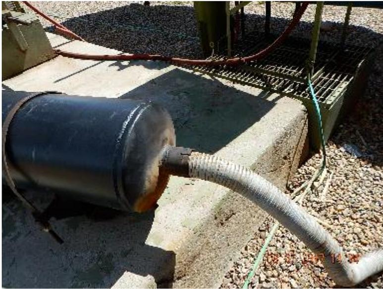
Photo 15: Flex pipe connection at back of in-line muffler.
