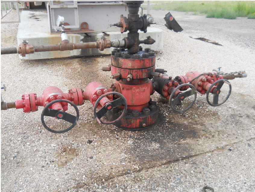
Stained soil south side of wellhead looking north. Draining off of pump jack skid as well
