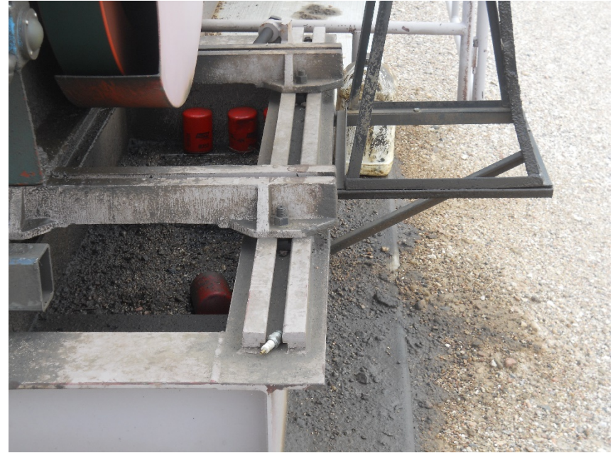
Stained soil northwest side of pump jack. Trash needs picked up
