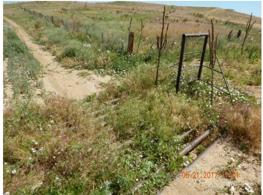
Photo 2. Photo taken from the just west of the meter shed, facing North. Operator needs to remove the cattle guard from location. As of August 10, 2017, the cattle guard still remains at location.
