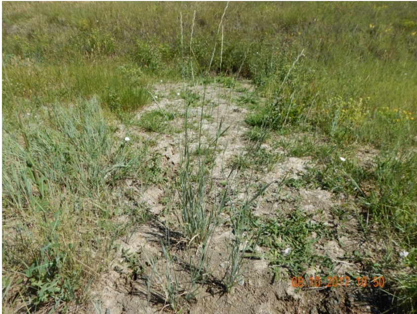
Photo 2. Photo taken from Culvert #2, facing North. Culvert has been removed and disturbance area seeded. No stormwater erosion was observed.
