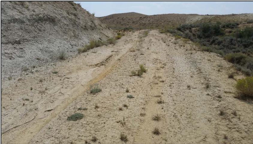
**Photo 3. Erosion on access road.**
