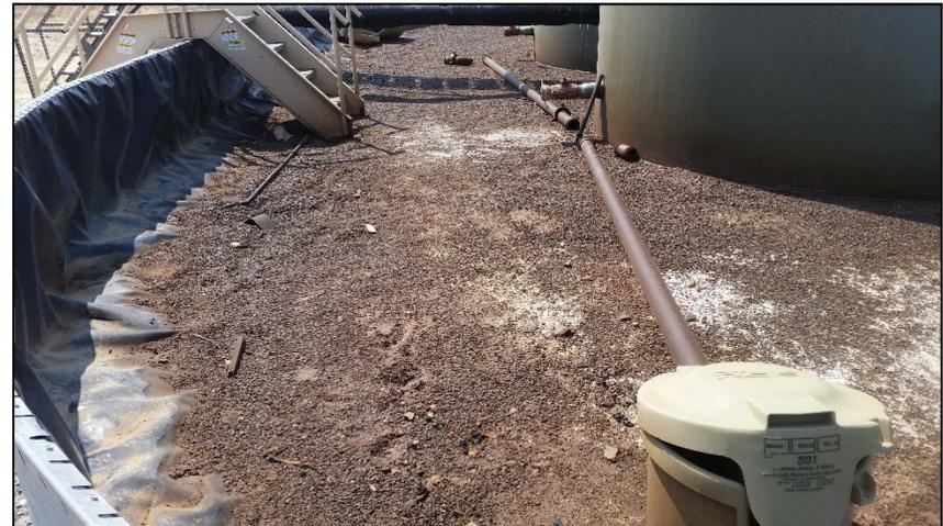
**Photo 2. Stained material from spill remains in berm.**
