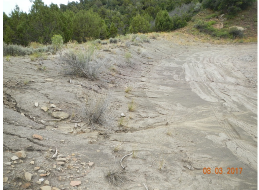
Photo 2: View of the eastern portion of the project area from the northeastern corner of the well pad facing southward. This slope is not stabilized and is eroding.
