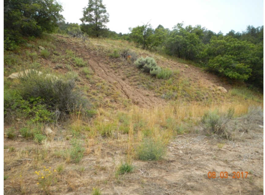
Photo 6: View of the southern portion of the project area from the eastern edge facing southwestward. Rilling is occurring on the cut-slope.
