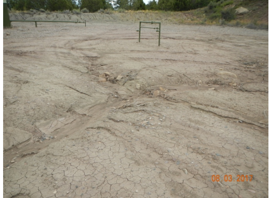
Photo 4: View of erosional channel in the northern portion of the project area, approximately 2 feet wide and 8 to 12 inches deep, facing upstream onto the well pad.
