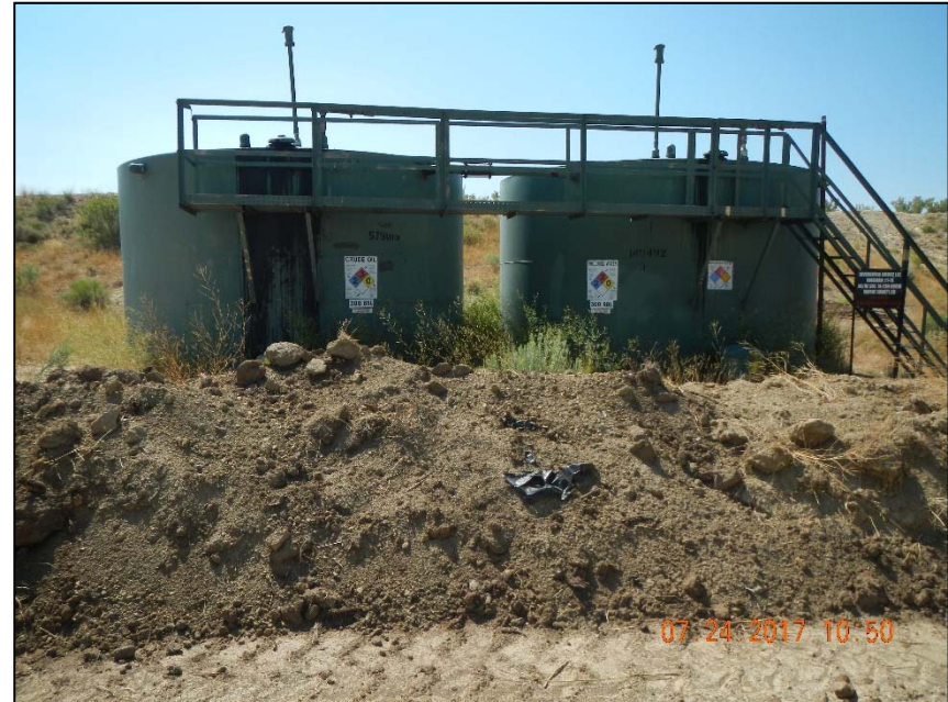
Photo 2. Unconsolidated berm with plastic liner pieces mixed in. Weeds in berm.
