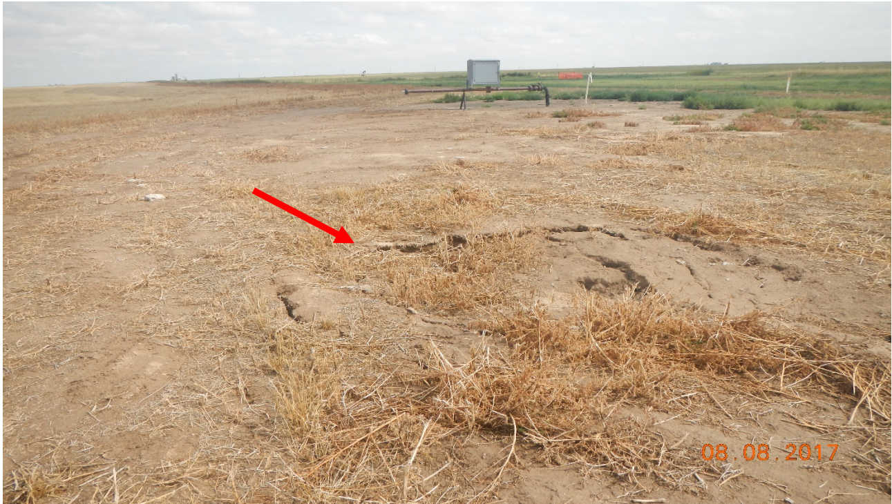
photo 3: The arrow points to an area of subsidence beginning to occur.
