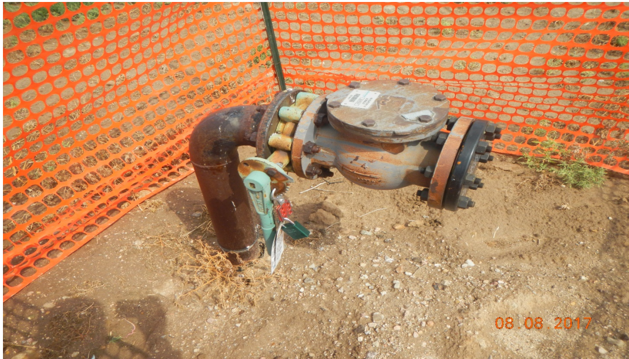
photo 3: The riser is locked and tagged out.
