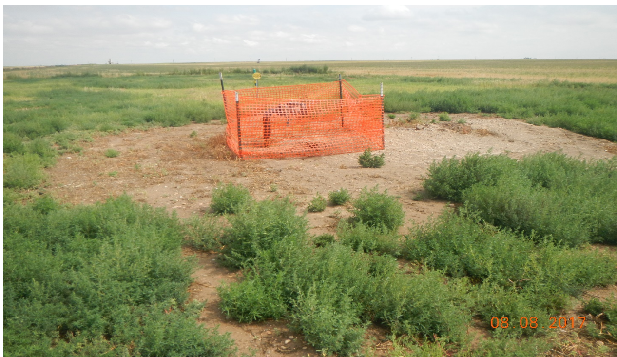
photo 2: There is a pipe riser that remains at the former battery site Lat/Long:39.84499,-104.45152. It appears to have been disassembled since previous inspection however, riser still remains.
