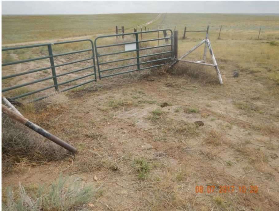
Photo 7: Photo taken from access road, east of the location. Inspection doc. #682501867 required operator to removed cattle guard. Photo shows cattle guard that has not been removed.
