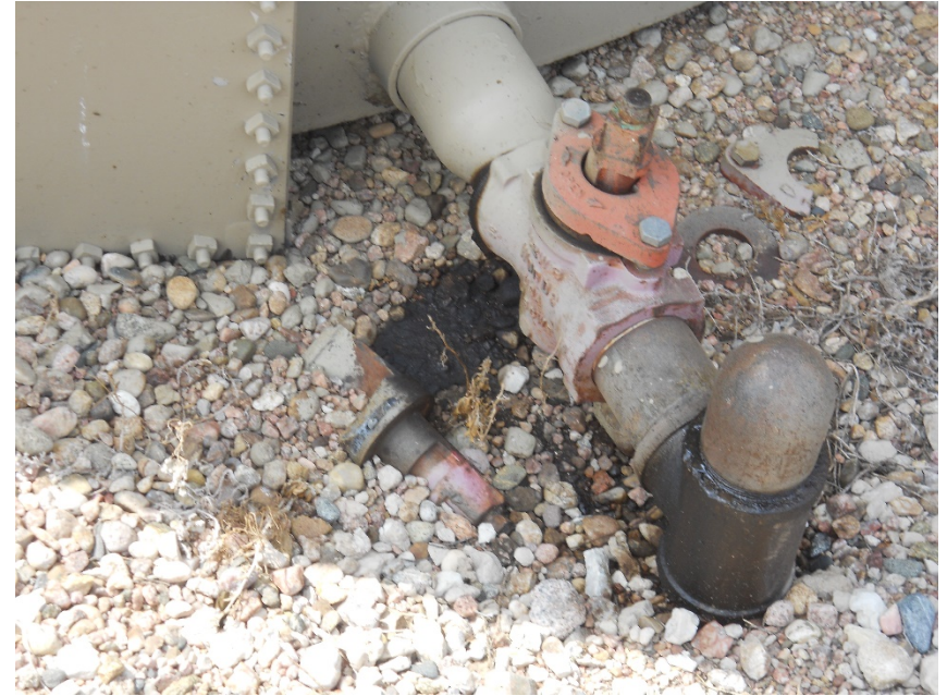
Backside valve of west crude tank, stained soil
