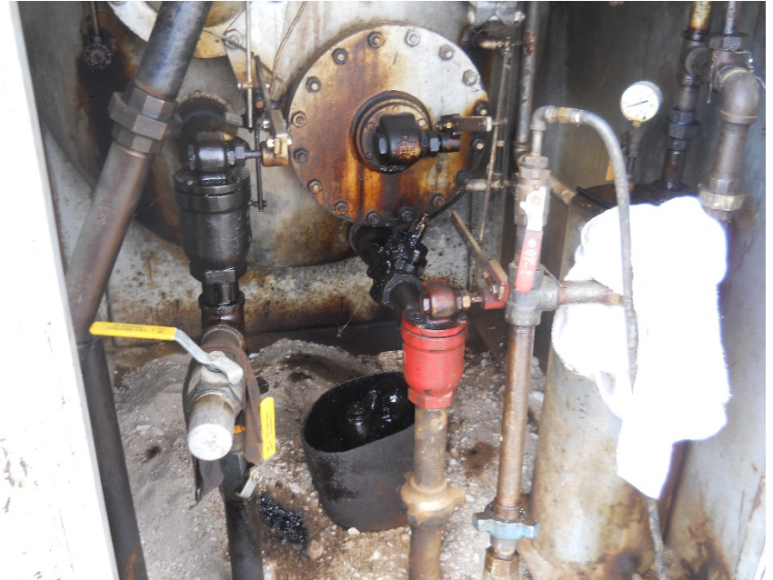
Leaking valves and stained soil inside of separator dog house
