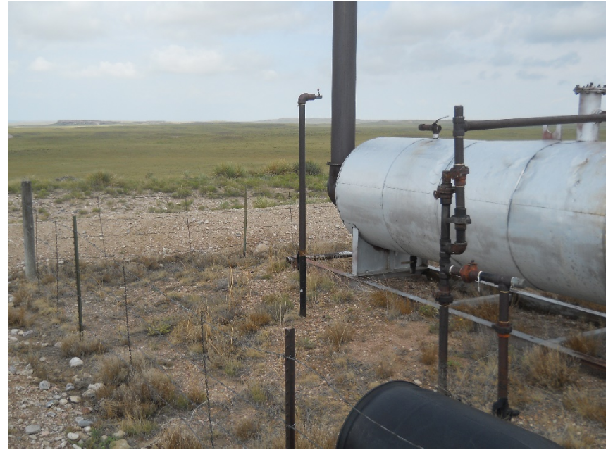
2" Unused/unmarked riser on south side of separator
