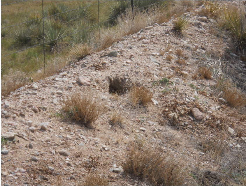
Animal burrow inside of berm on west side of tank battery
