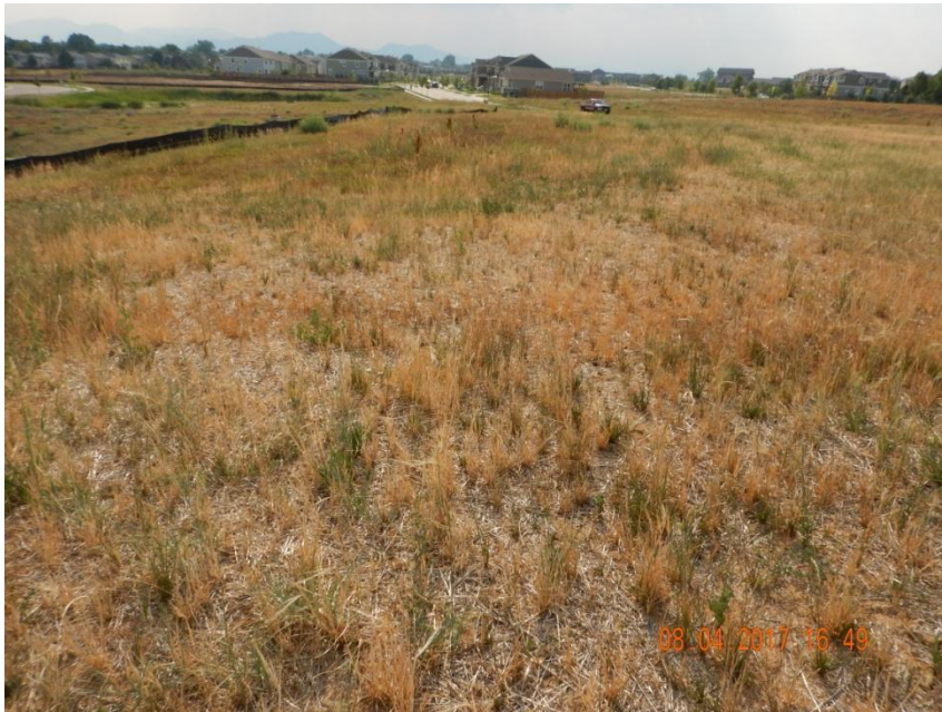
Photo 3. Photo taken from the southern location, facing West. Location appears to be sufficiently stabilized with vegetation and straw mulch until the location is further developed into housing development. Silt fence BMP has been installed along the down gradient eastern and southern location as well.
