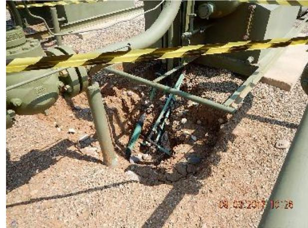
**Photo 8: Excavated 1" line at separator. Valve inside cabinet is locked out and painted.**
