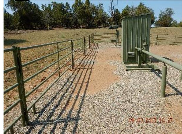
**Photo 10: Sediment deposits inside fenced production equipment area.**
