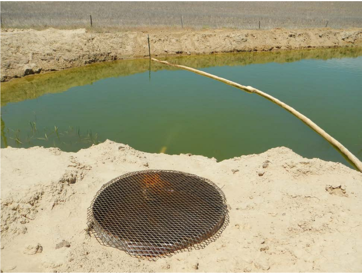
Final skimmer prior to discharge into western produced water pit.
