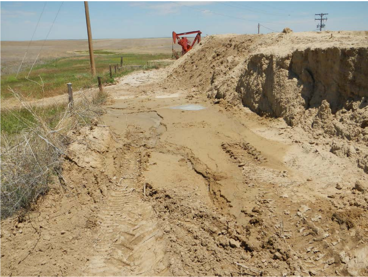
View north along west side of produced water pit.
