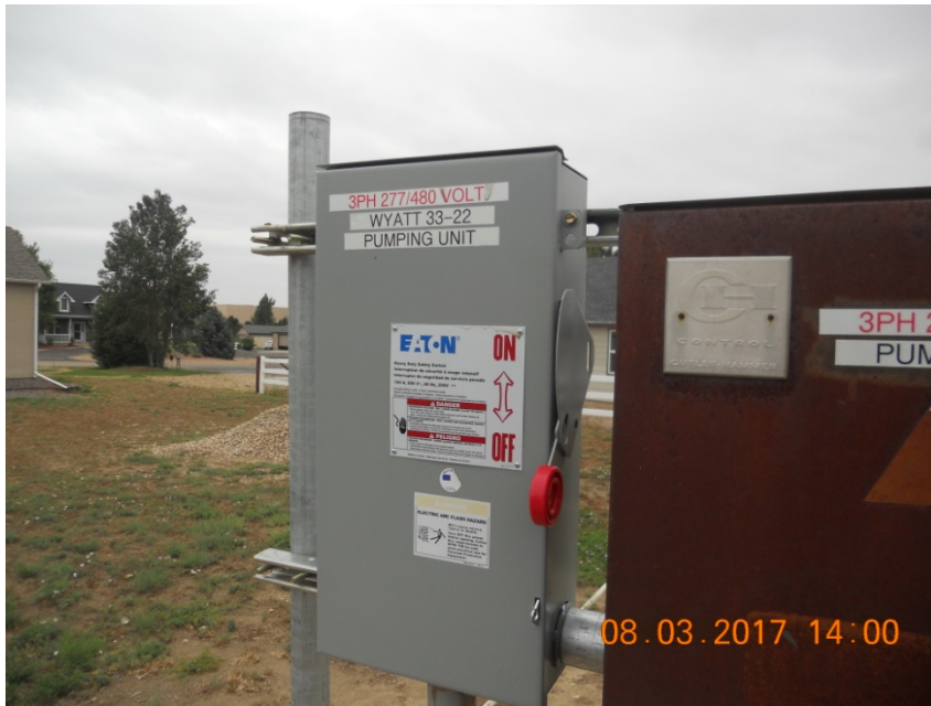
Photo 3. Electrical disconnect for Wyatt 33-22 at electrical panel station
