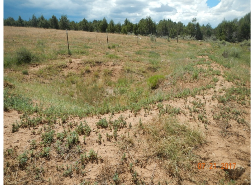
Photo 4: View of sediment trap near the well pad entrance that appears to be functioning.
