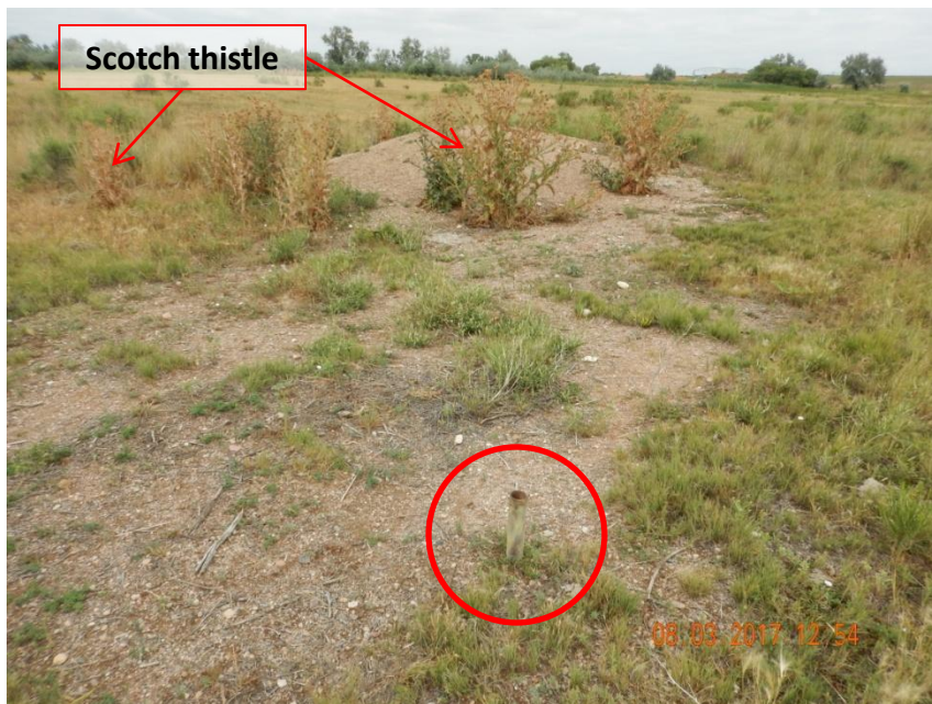
Photo 1. Photo taken from the well location, facing North. Location does not meet Rule 1004 standards. Gravel pile and gravel remains at the well location, and noxious weeds were observed. Well marker does not comply with Rule 319.a.(5).
