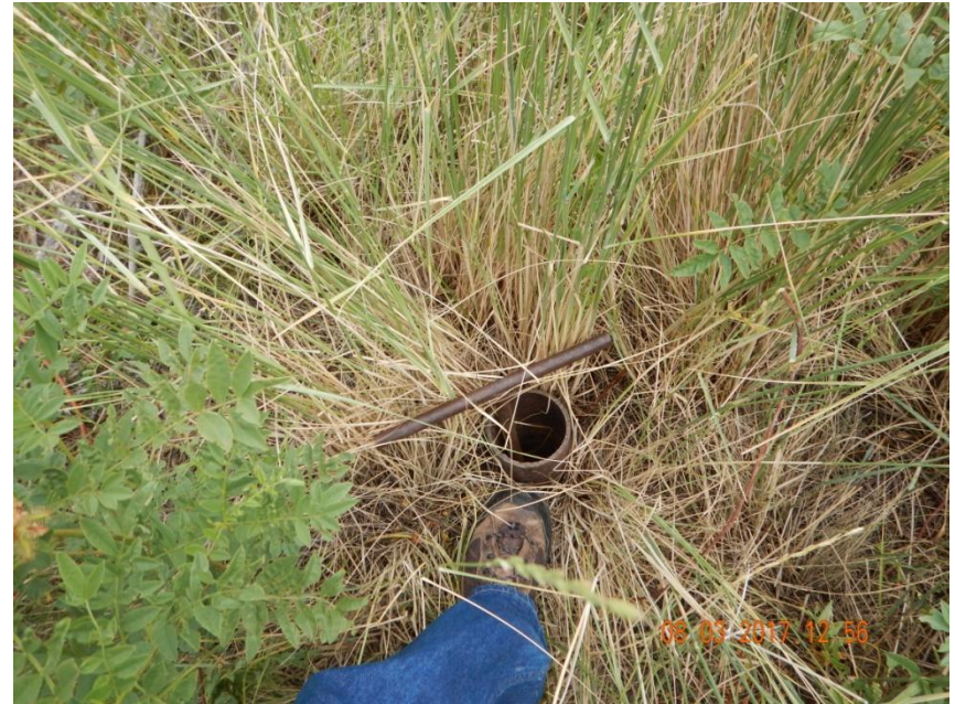
Photo 4. Close-up photo (2 of 2) taken of some of the pipe risers at location.
