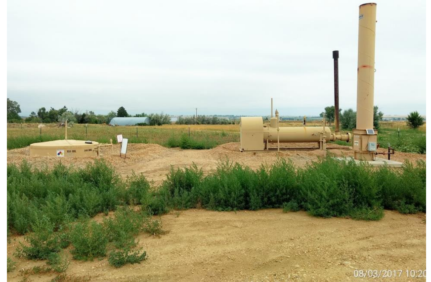
Separator, water tank, & ECD, Corrective action: Overgrown weeds.
