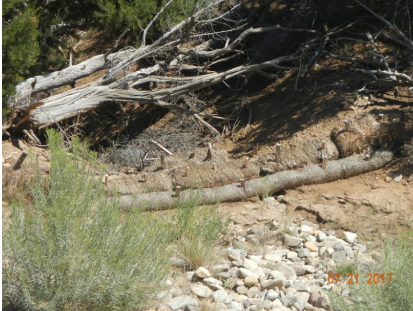
Photo 5: View of wattles along the eastern edge of the well pad where stormwater is flowing beneath the wattle and needs maintenance.
