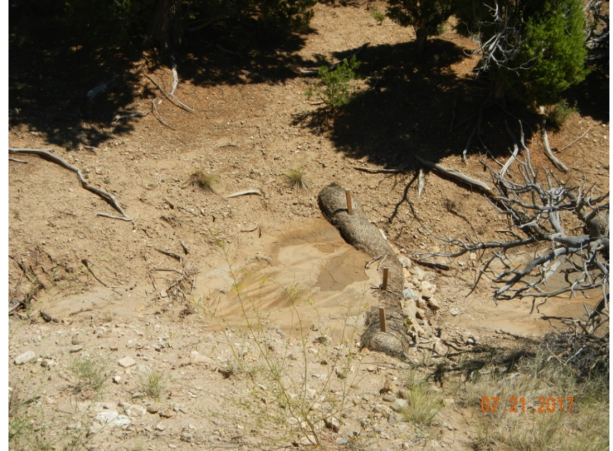
Photo 4: View of wattle on the northeastern edge full of sediment that needs maintenance.
