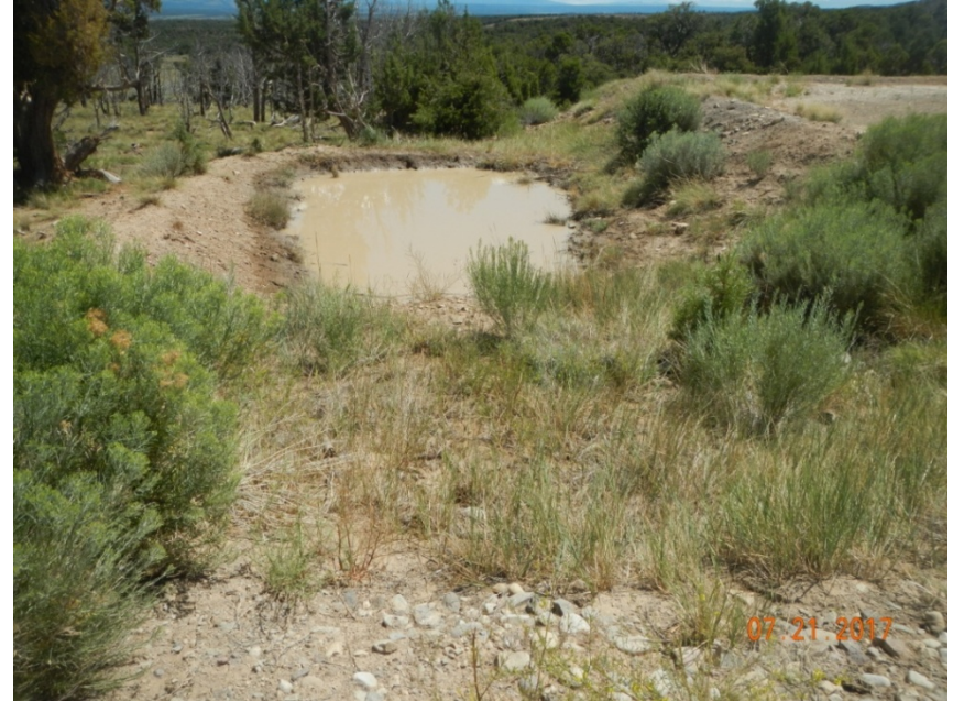
Photo 6: View of sediment trap east of the well pad entrance.
