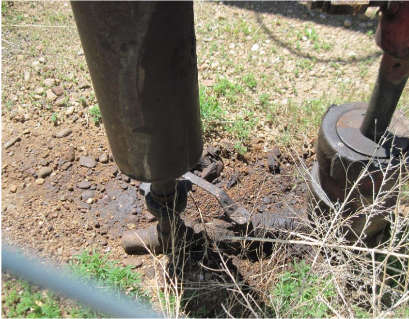
Wellhead, from 6/20/2017 inspection photos. Corrective action: Stained soil at wellhead
