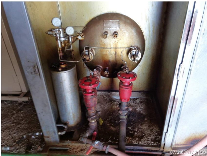
Inside of separator housing, Corrective Action: Stained soil inside of separator cabinet
