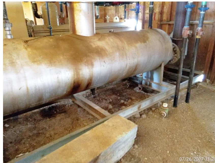
Inside of separator housing, Corrective action: Stained soil at separator. Note Unidentified riser.
