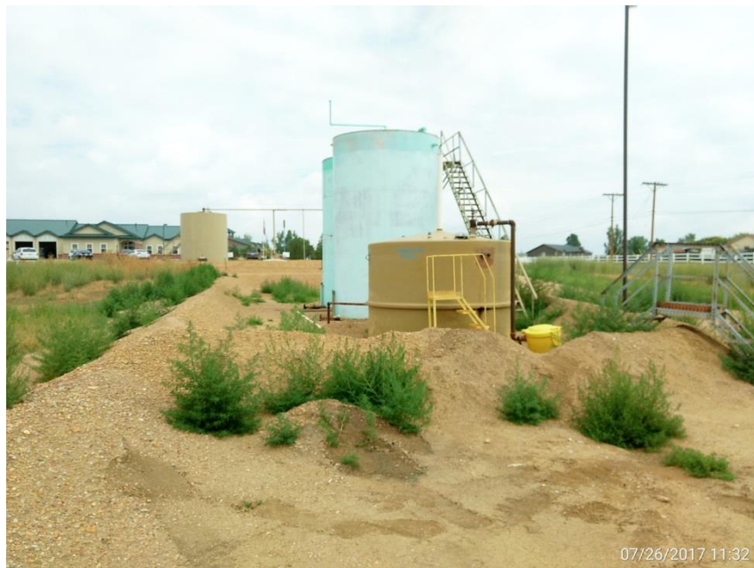
Tank battery, Corrective Action: Berm maintenance and weeds.
