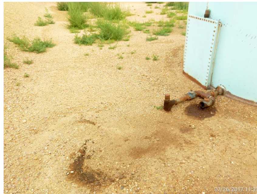
Inside of oil/water tank berm, Corrective Action: stained soil and weeds.
