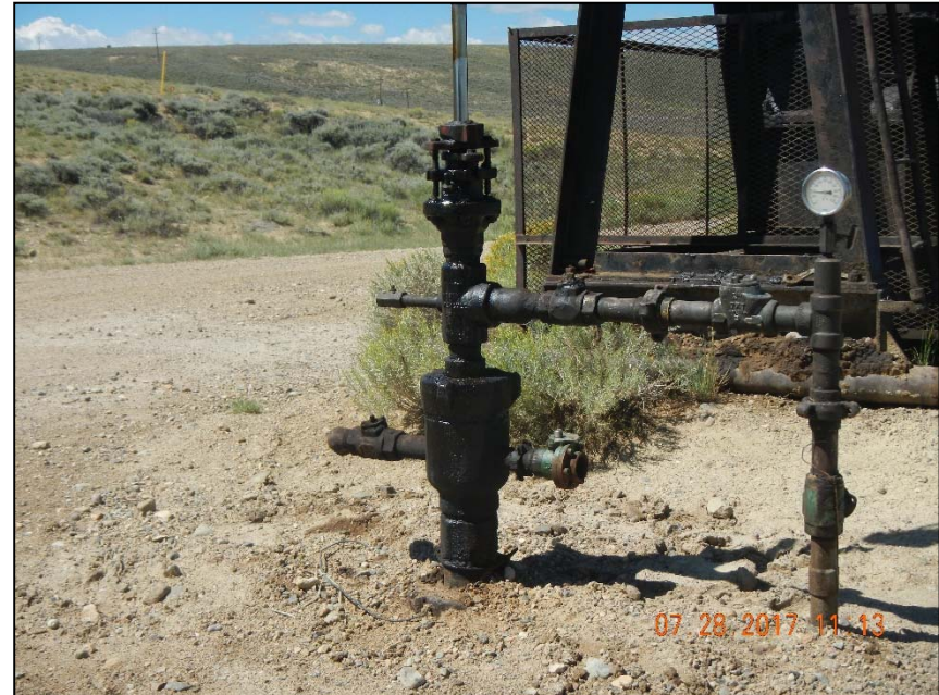
Photo 2. Leak at wellhead.
