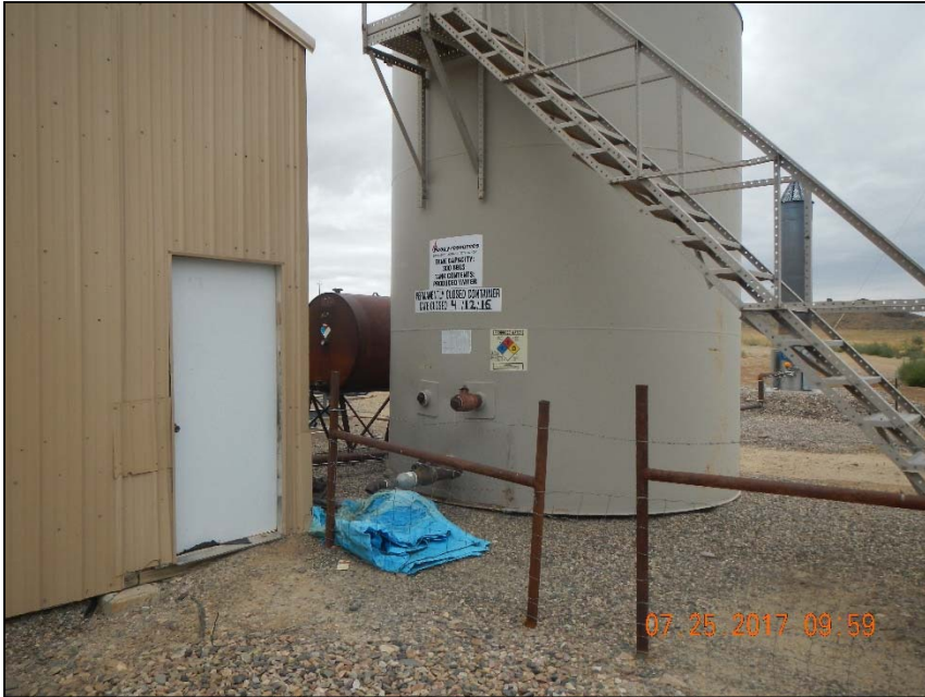
Photo 2. Produced water tank marked out of service stored on location.
