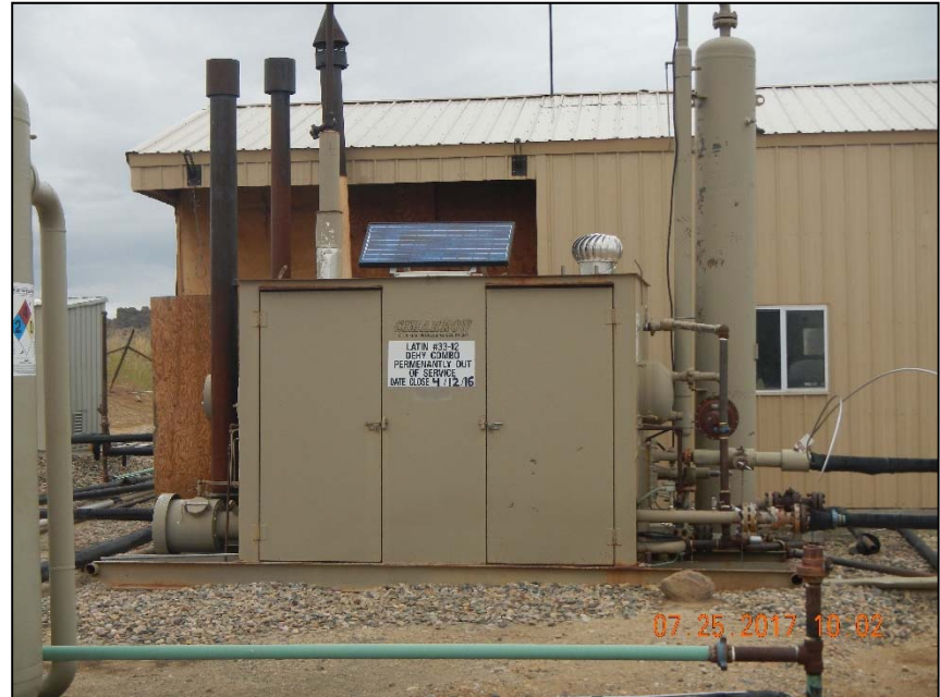
Photo 3. Seperator treater marked out of service stored on location.
