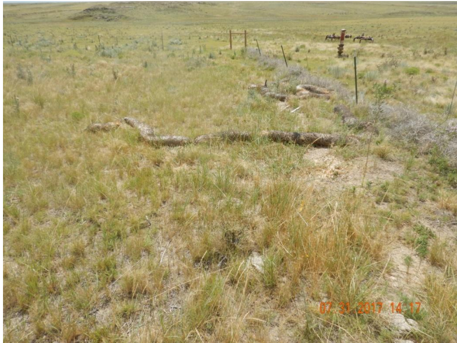
Photo 3: Photo taken from the location. Photo straw wattles on location. Wattles were likely used as a stormwater BMP, however wattles have not been maintained and are now debris.
