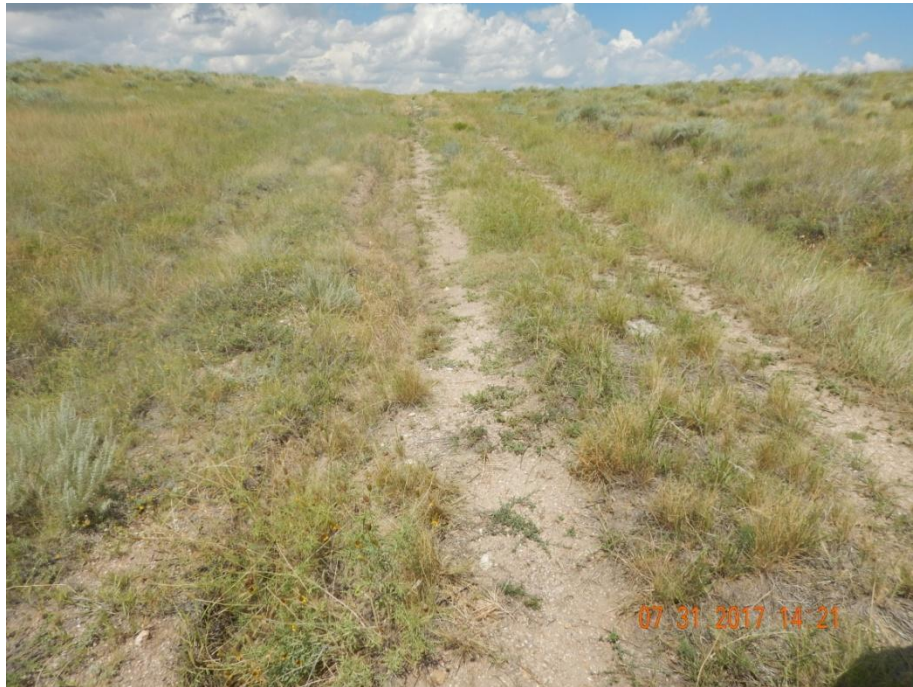
Photo 7: Photo taken from the access road on the north end of the location, facing north. Photo shows access road has not been re-contoured or re-graded.
