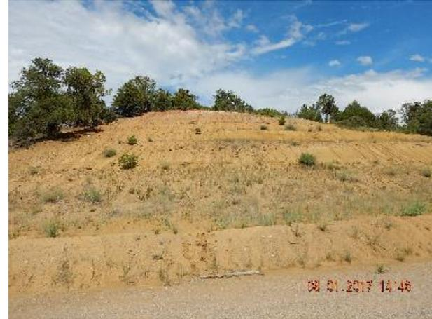
Photo 4: Rilling and storm water overrun at bottom of cut slope.
