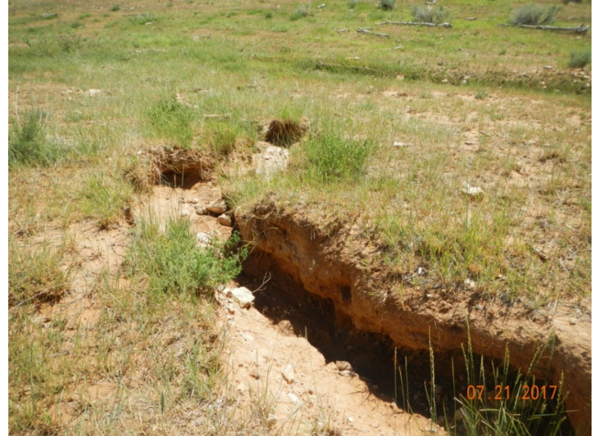
Photo 4: View of diversion that is eroding in the southeastern portion of the project area, that feeds to the silt trap in Photo 5. Stormwater controls should be applied to de-energize flows in this diversion.
