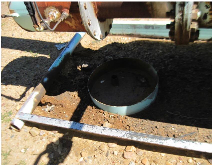
Separator, from 6/20/2017 inspection, Corrective action: stained soil.
