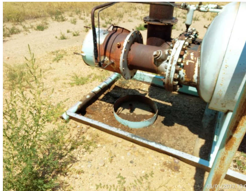
Separator fire tube, Corrective action: stained soil not remediated.
