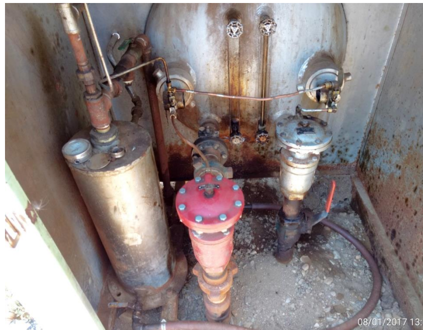
Separator cabinet, Corrective action: Stained soil, leaking dump line.
