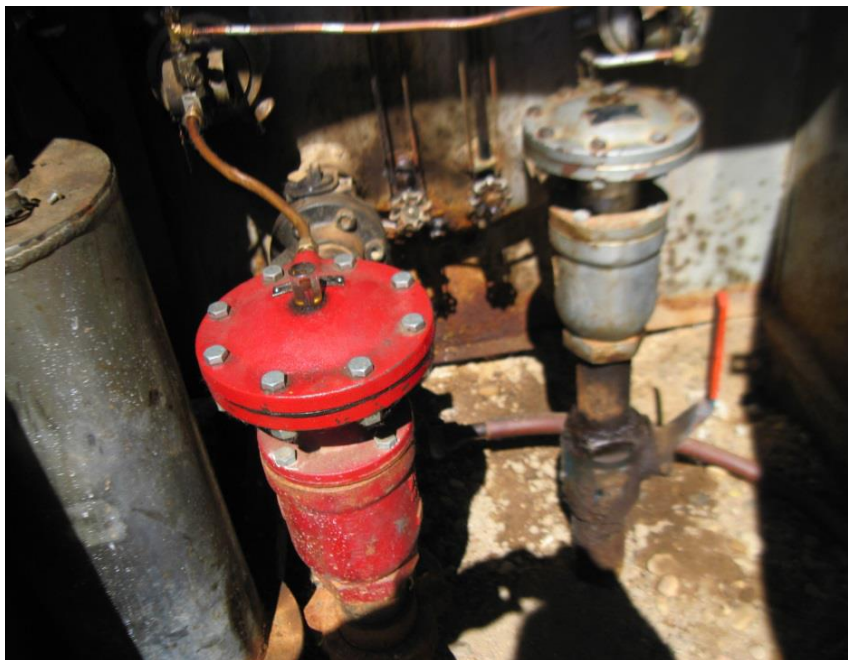
Separator cabinet from 6/20/2017 inspection, Corrective action: stained soil, leaking dump line.
