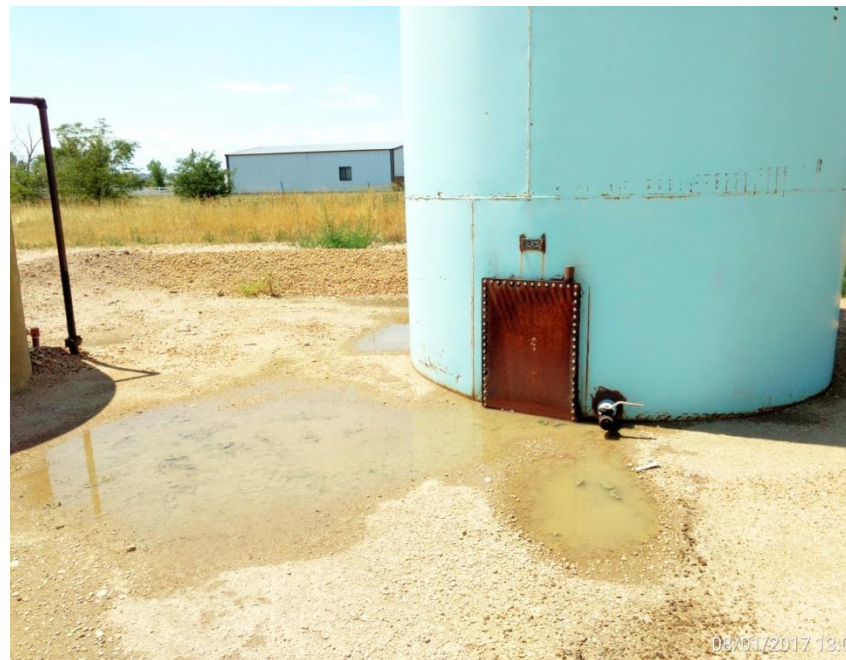
Inside oil/water tank berm, Corrective action: Stained soil not remediated.
