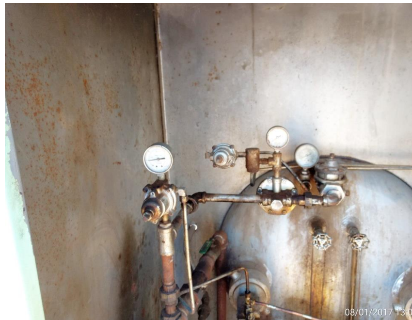
Separator cabinet, audible leak on scrubber pot, note pressure gauge.
