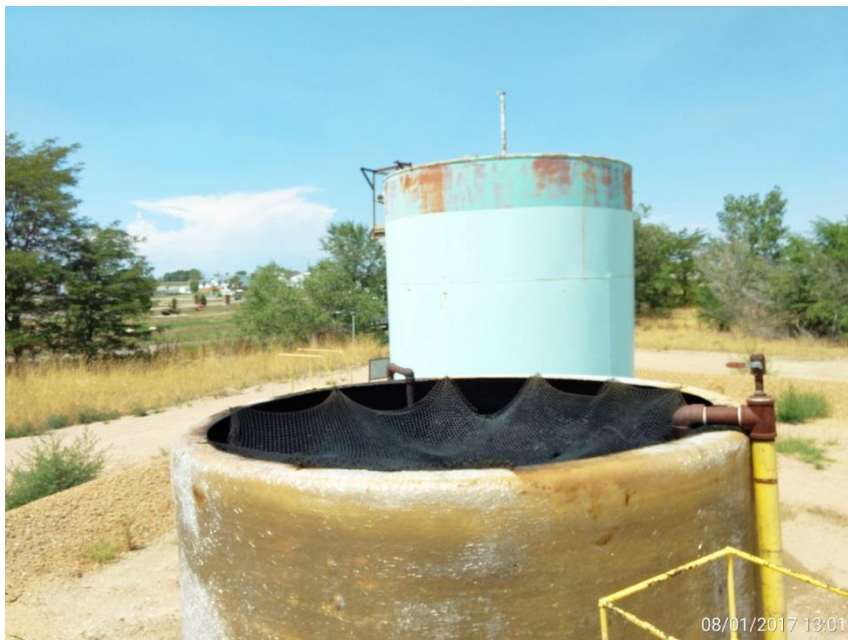
Water tank, Corrective action: netting on open top ineffective.
