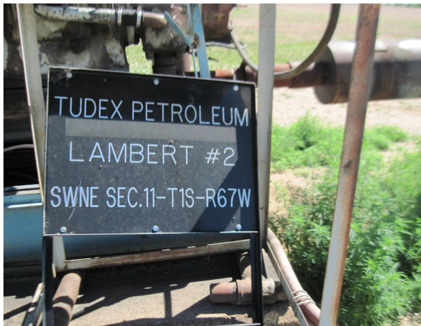
Wellhead signage from 6/20/2017 inspection, Corrective action: No emergency contact info.
