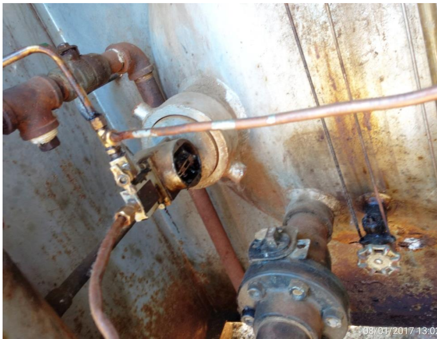
Separator Cabinet: Corrective action: Visible leak on dump valve
