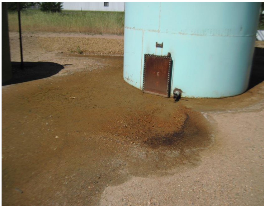
Inside oil/water tank berm, from 6/20/2017 inspection, Corrective action: Stained soil.
