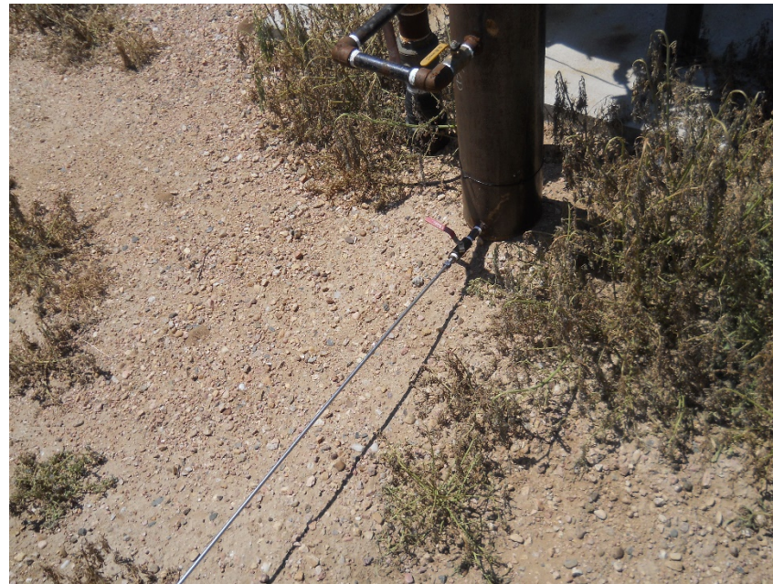
6) Scrubber drain on north ECD plumbed through fence
