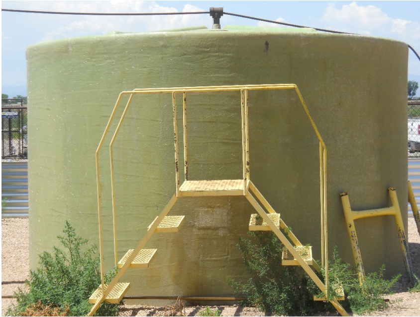
17) Weeds inside of berm, no signage on water tank labeling contents, capacity, NFPA label
