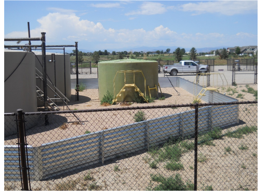
10) Weeds inside of tank battery looking west, no water tank signage
