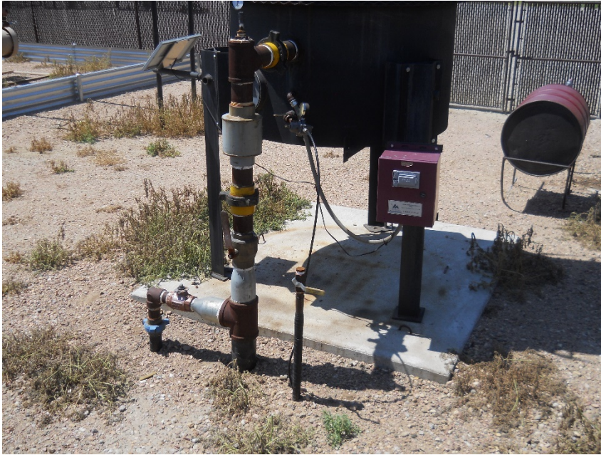
9) Unmarked/unused 1" steel riser at south ECD
