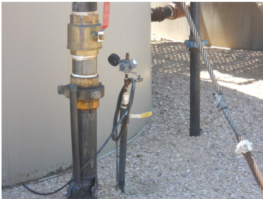
15) Unmarked/unused 1" steel riser next to northeast tank
