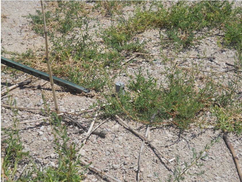
21) Unmarked anchor on northwest corner of location
