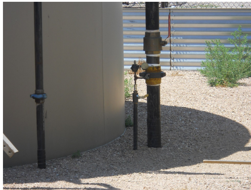
16) Unmarked/unused 1" steel riser next to northwest tank
