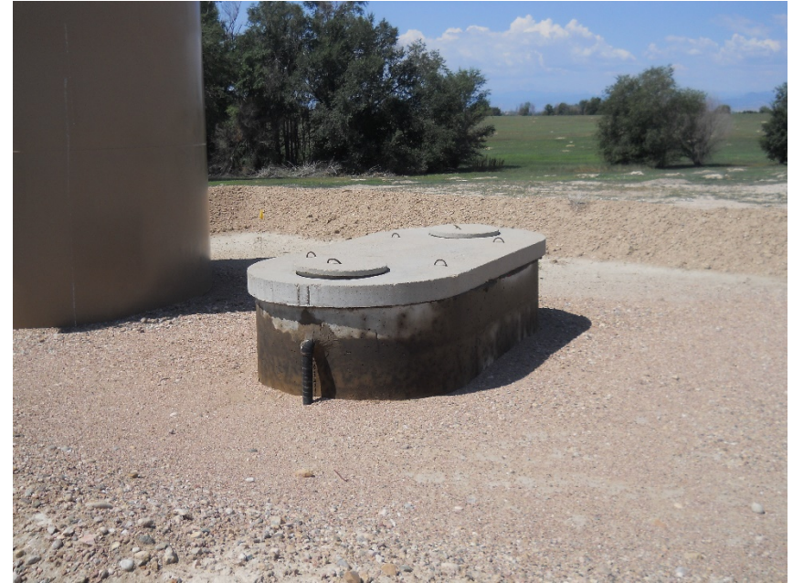
6) Water vault looking west. No contents, capacity, or NFPA label
