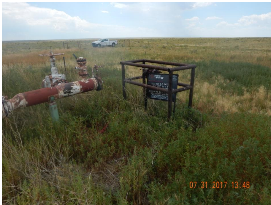
Photo 3: Photo taken from the location. Photo shows pipe riser equipment remains on the location.
