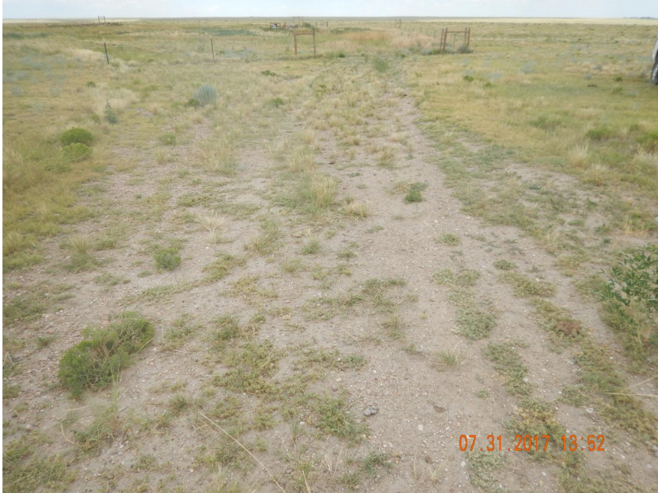
Photo 7: Photo taken from the access road, facing north. Gravel remains evident at access road, and road remains predominantly unvegetated and does not meet reclamation requirements.
