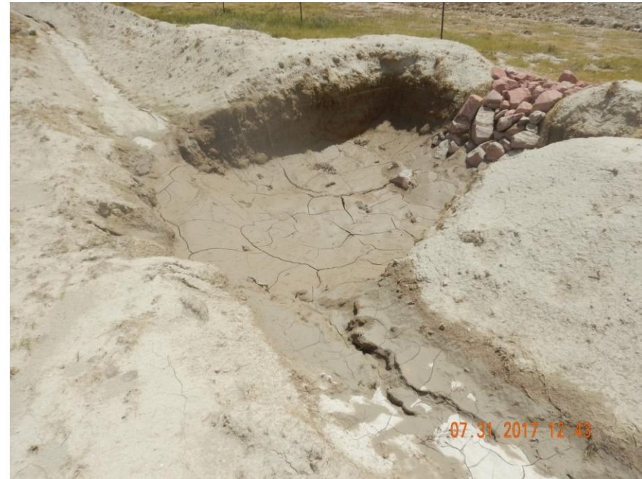
Photo 4: Photo taken from the south end of the location. Photo shows sediment trap. Photo shows stormwater erosion has begun to erode at the inlets of the trap. Sediment does not appear to have sufficient inlet protection.
