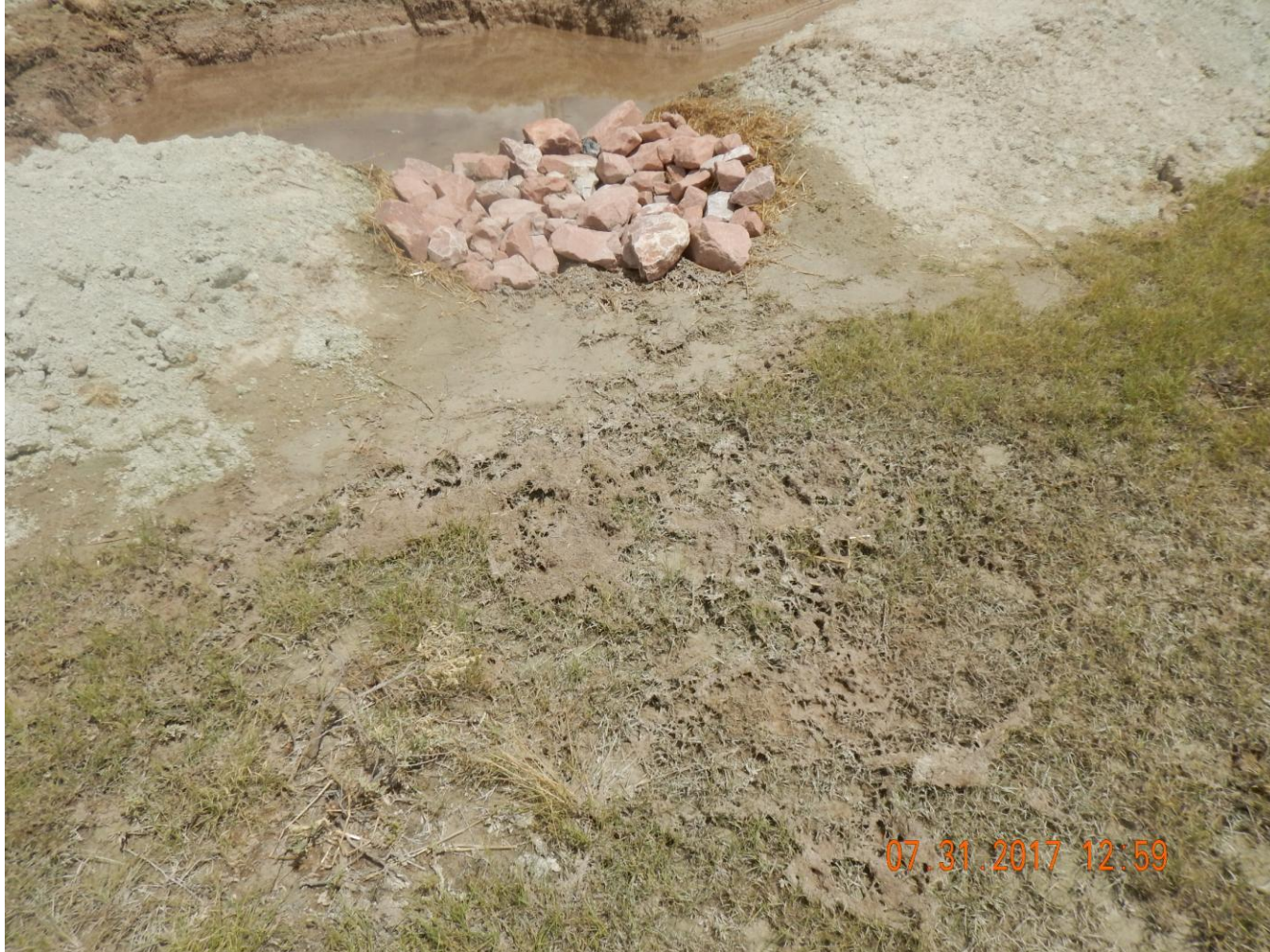
Photo 19: Photo taken from the sediment trap on the southwest corner of the location. Photo shows sediment laden stormwater has discharged from the location. Trap does not appear to have sufficient outlet protection.
