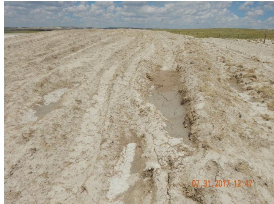
Photo 10: Photo taken from the topsoil pile on the east end of the location. Photo shows topsoil pile is loose, and does not appear to have sufficient protection; pile appears to be at risk to stormwater and wind erosion.
