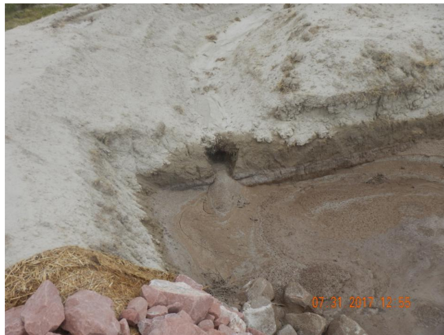
Photo 16: Photo taken from the northwest end of the location. Photo shows sediment trap. Photo shows stormwater erosion has begun to erode at the inlets of the trap. Sediment does not appear to have sufficient inlet protection
