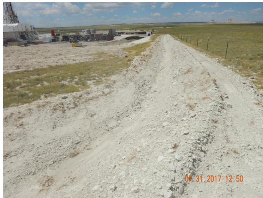
Photo 12: Photo taken from the northeast end of the location, facing south. Photo shows stormwater control ditch along perimeter of the location.
