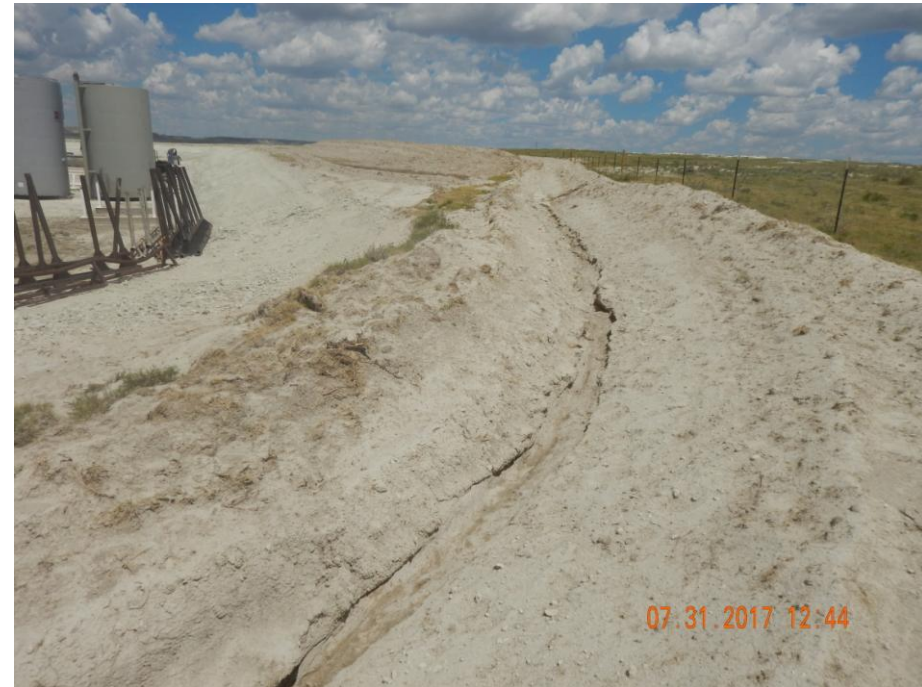
Photo 6: Photo taken from the southeast end of the location, facing north. Photo shows stormwater control ditch along perimeter of the location. Photo also shows stormwater erosion has begun to incise the perimeter ditch. Advise incorporating velocity check BMPs to mitigate further incision and degradation to the ditch.
