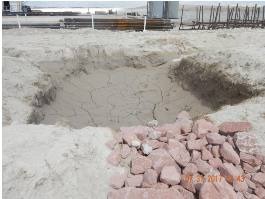
Photo 3: Photo taken from the south end of the location. Photo shows sediment trap. Trap appears to either have filled with sediment, or constructed with a shallow depth.
