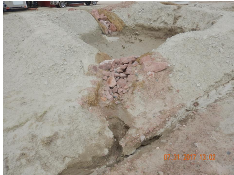
Photo 21: Photo taken from the south end of the location (west of cattle guard). Photo shows sediment trap. Photo shows stormwater erosion has begun to erode at the outlet of the trap, contributing to sediment laden stormwater discharge.. Sediment does not appear to have sufficient outlet protection.
