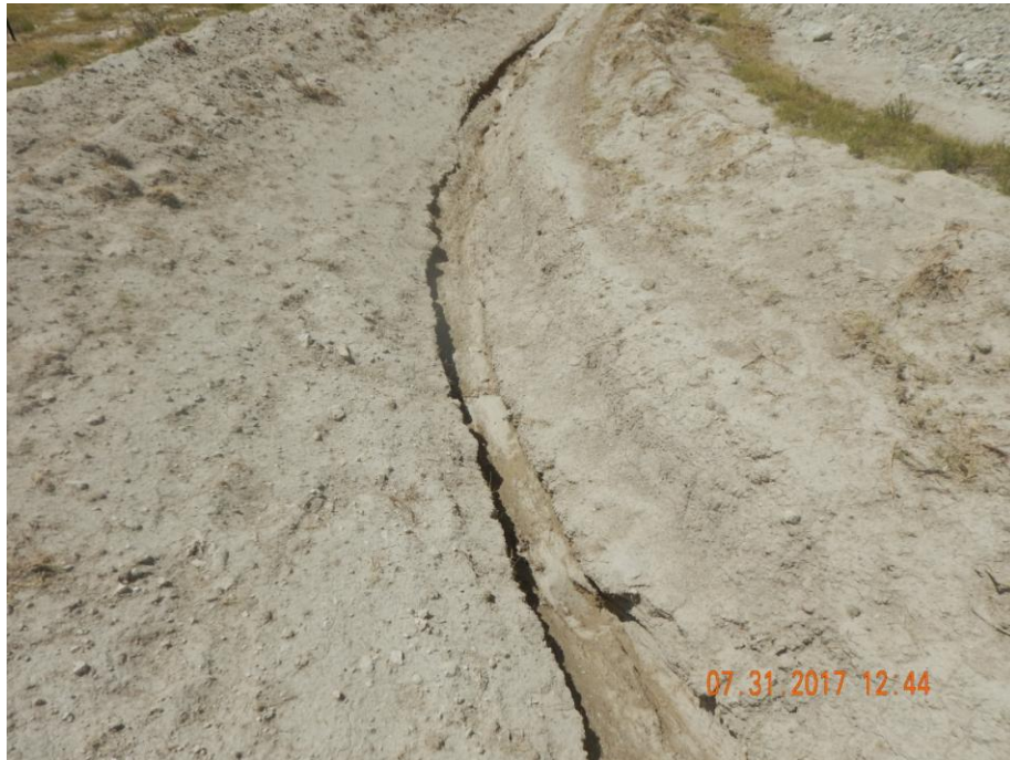
Photo 9: Photo taken from the stormwater control ditch on the east end of the location. Photo shows stormwater erosion has begun to incise the perimeter ditch. Advise incorporating velocity check BMPs to mitigate further incision and degradation to the ditch.
