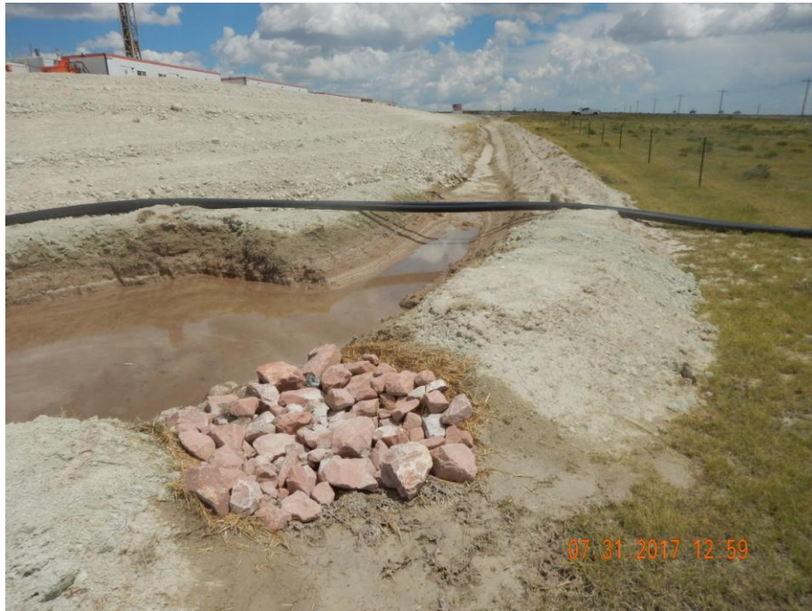
Photo 17: Photo taken from the southwest end of the location, facing east. Photo shows sediment trap and stormwater control ditch.
