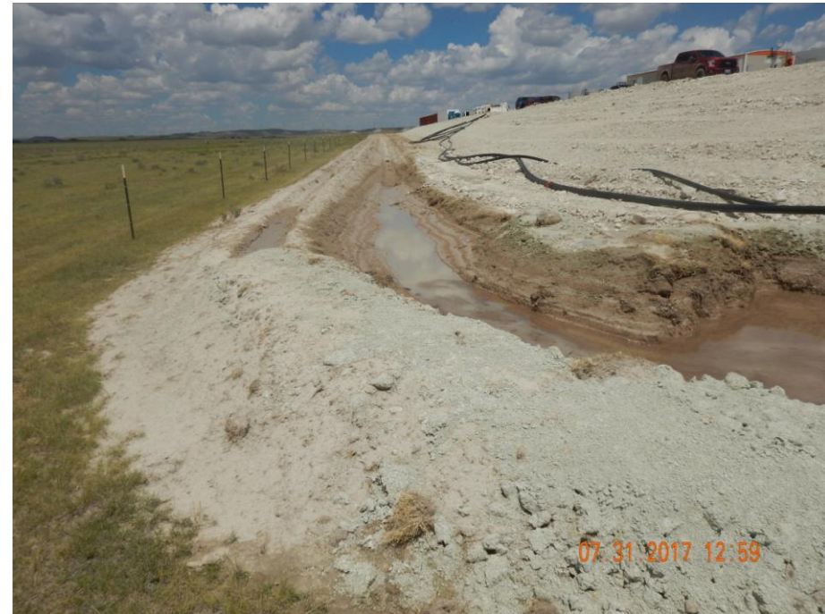
Photo 18: Photo taken from the southwest end of the location, facing north. Photo shows sediment trap and stormwater control ditch.
