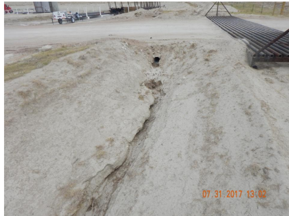
Photo 2: Photo taken from the south end of the location, facing east. Photo shows the west end of the culvert at the access road. Photo shows stormwater erosion has begun to incise the perimeter ditch at the culvert. Culvert does not appear to have sufficient outlet protection.
