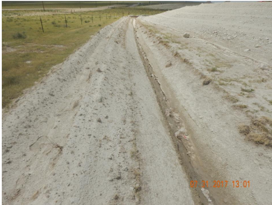
Photo 20: Photo taken from the stormwater control ditch on the east end of the location. Photo shows stormwater erosion has begun to incise the perimeter ditch. Advise incorporating velocity check BMPs to mitigate further incision and degradation to the ditch.
