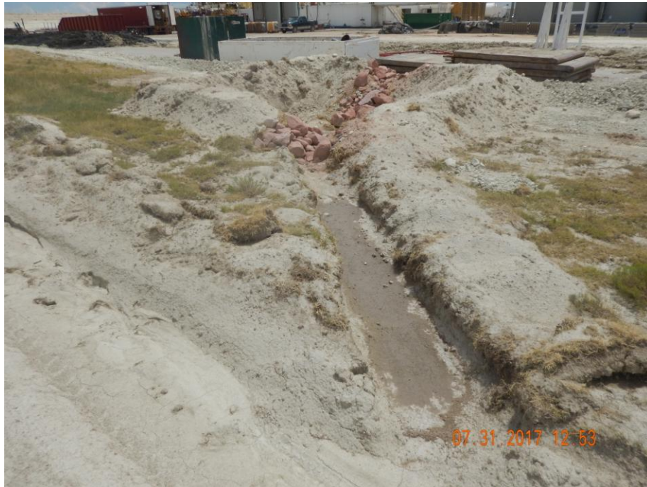
Photo 13: Photo taken from the north end of the location. Photo shows sediment trap outlet. Sediment appears to be in proper functioning condition.
