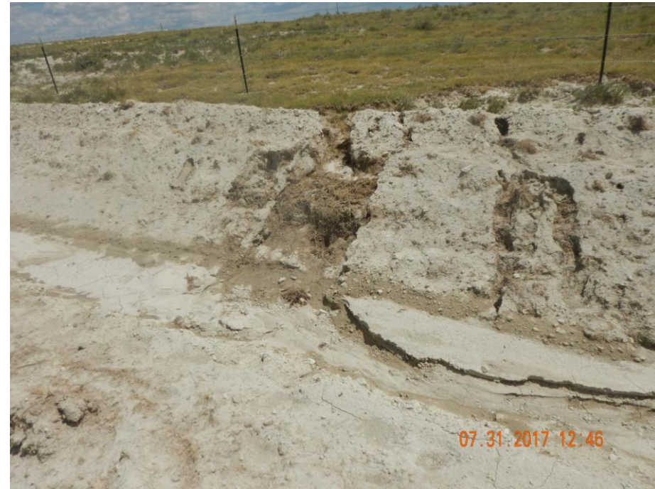
Photo 8: Photo taken from the storm water ditch on the east end of the location. Photo shows stormwater erosion has compromised the integrity of the ditch. Ditch does not appear to have been sufficiently consolidated. Without adequate consolidation, ditch will increase the sediment laden stormwater runoff from the location.
