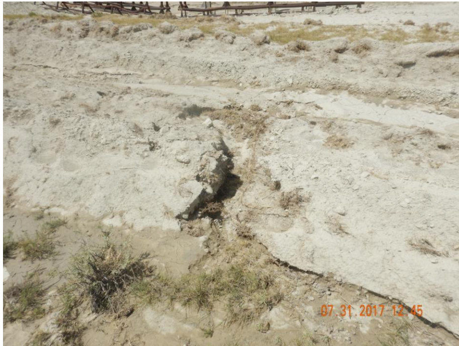
Photo 7: Photo taken from the storm water ditch on the east end of the location. Photo shows stormwater erosion has compromised the integrity of the ditch. Ditch does not appear to have been sufficiently consolidated. Without adequate consolidation, ditch will increase the sediment laden stormwater runoff from the location.
