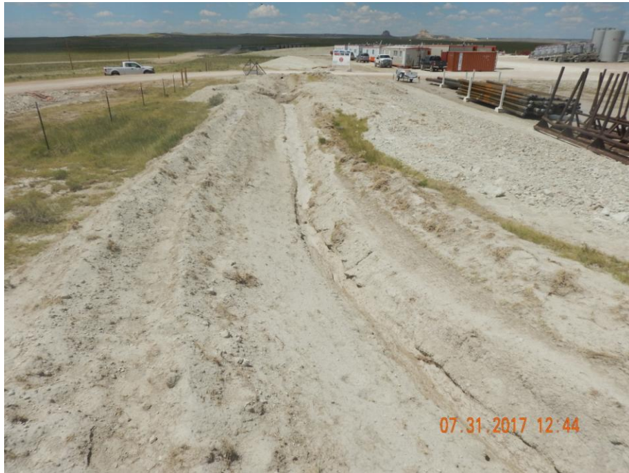
Photo 5: Photo taken from the southeast end of the location, facing west. Photo shows stormwater control ditch along perimeter of the location. Photo also shows stormwater erosion has begun to incise the perimeter ditch. Advise incorporating velocity check BMPs to mitigate further incision and degradation to the ditch.
