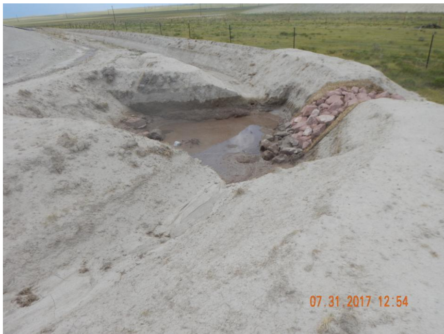
Photo 15: Photo taken from the northwest end of the location. Photo shows sediment trap.
