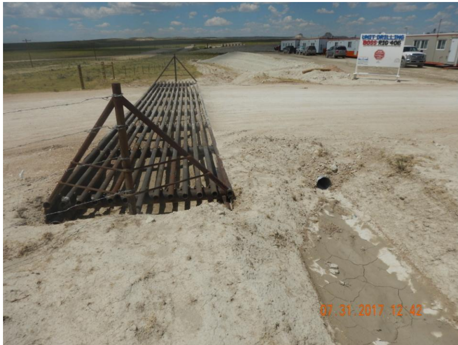
Photo 1: Photo taken from the south end of the location, facing west. Photo shows culvert and cattle guard.
