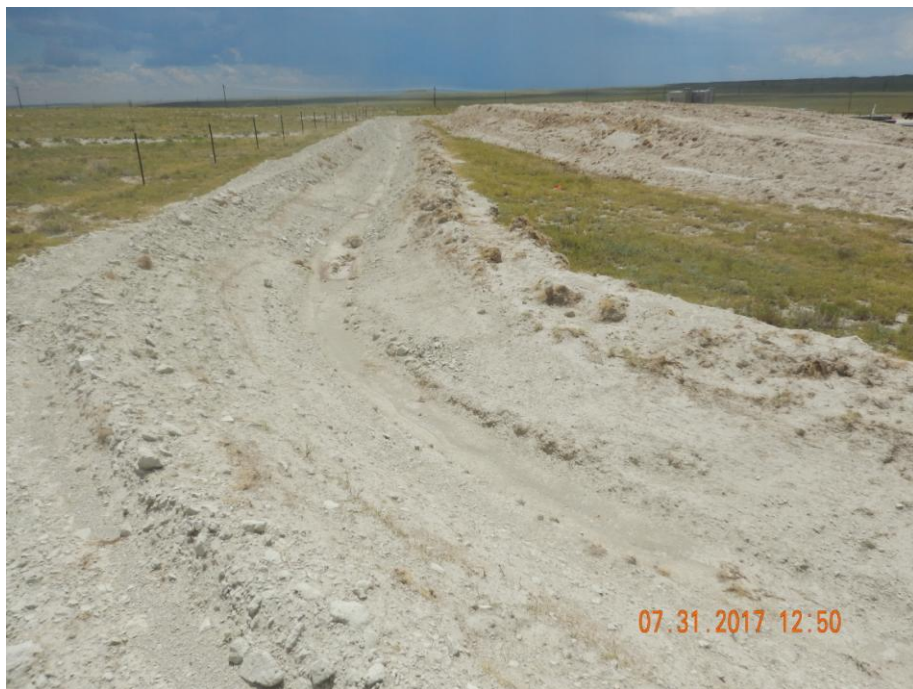
Photo 11: Photo taken from the northeast end of the location, facing south. Photo shows stormwater control ditch along perimeter of the location.
