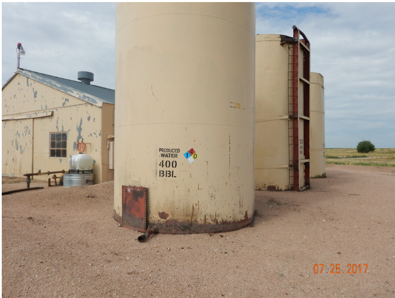
Figure 14 - Produced water ASTs on north side of injection plant (background).
