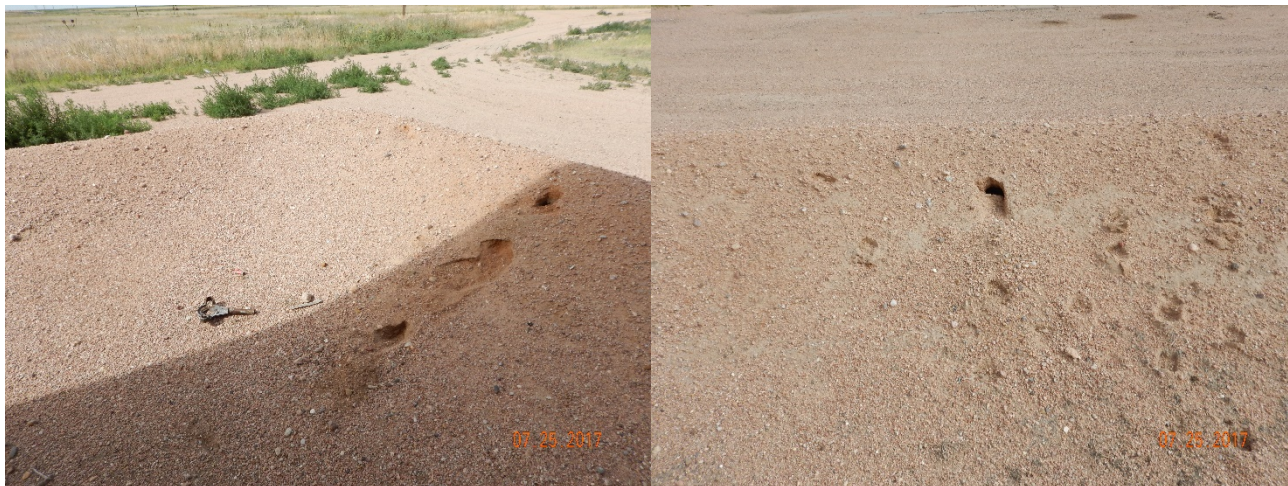
Figure 5 - Damaged earthen berms at crude oil ASTs.
