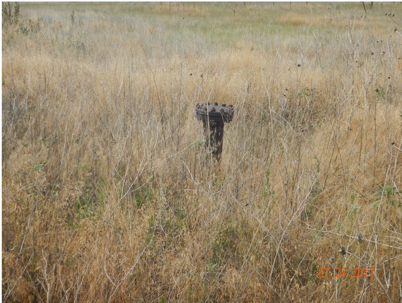
Figure 13 - Capped 8-12" riser south of crude oil ASTs.
