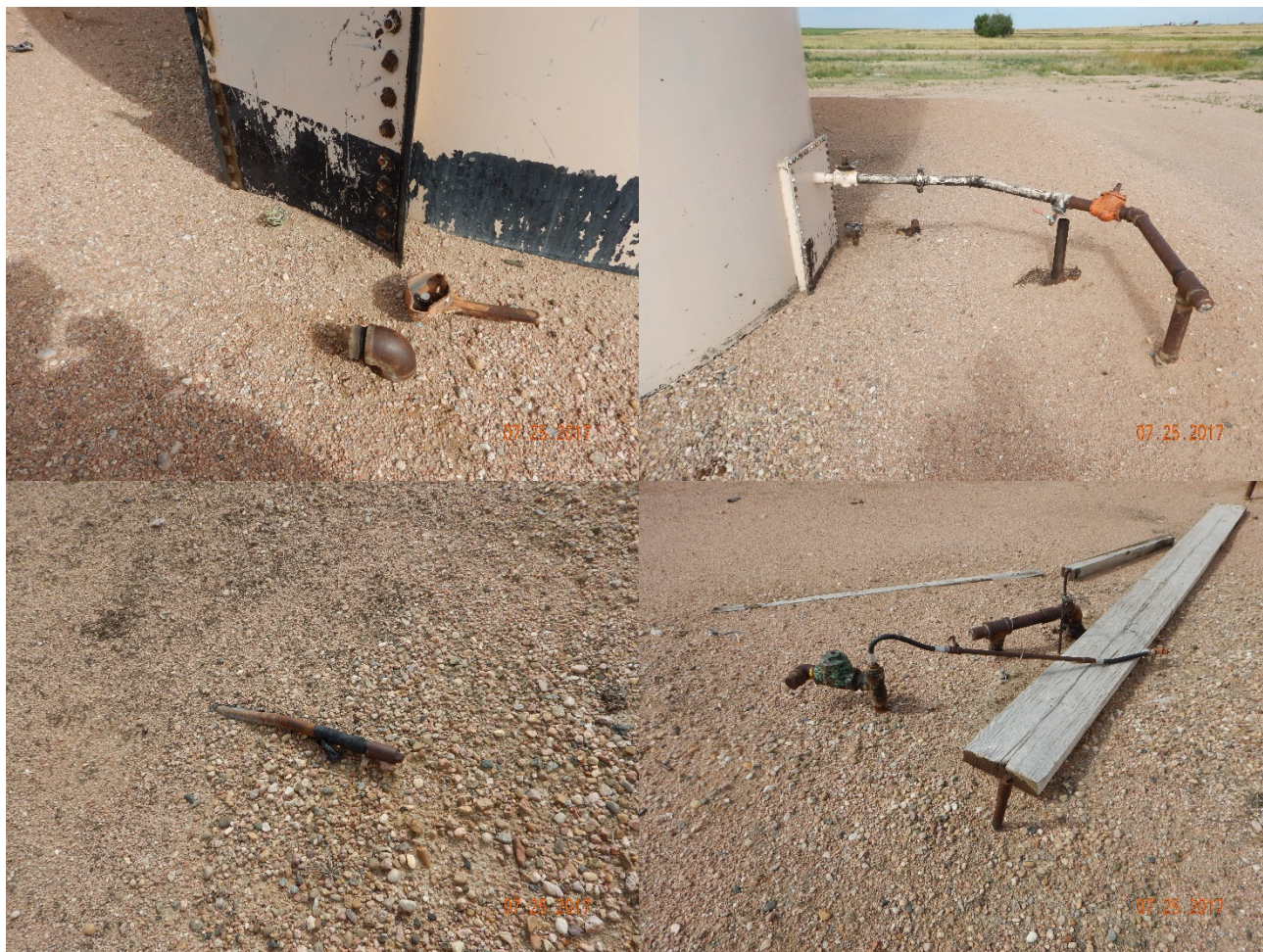
Figure 4 - Assorted flowline risers associated with crude oil ASTs.
