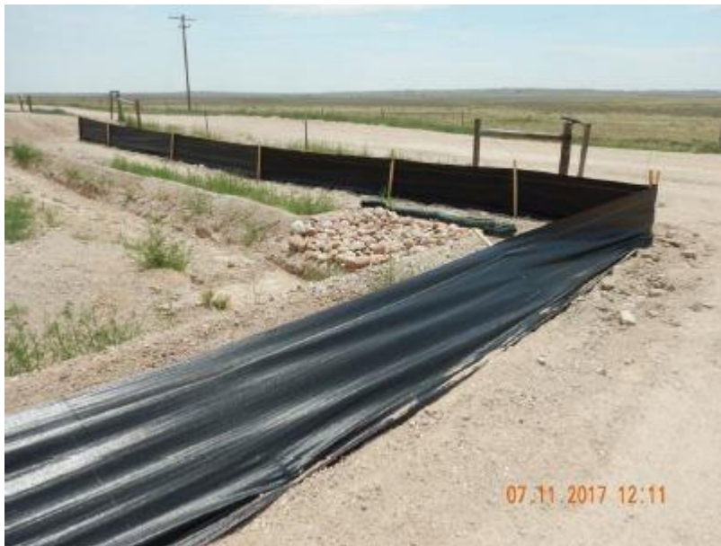
Photo 2. Photo taken from the southwest Holliday pad, facing Southeast. Silt fence BMP has not been properly installed. Silt fence is only pinned down and not buried/back-filled/compacted. Also, silt fence stakes should be installed to the outside of the silt fence, not inside of the silt fence
