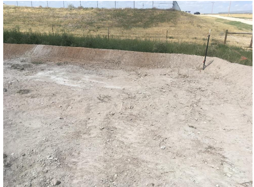
Photo NBL12. The berm has been repaired and re-compacted. Weeds have been mowed where accessible, and weeds have been sprayed site-wide. Hydromulch will be reapplied once the weeds have died.
