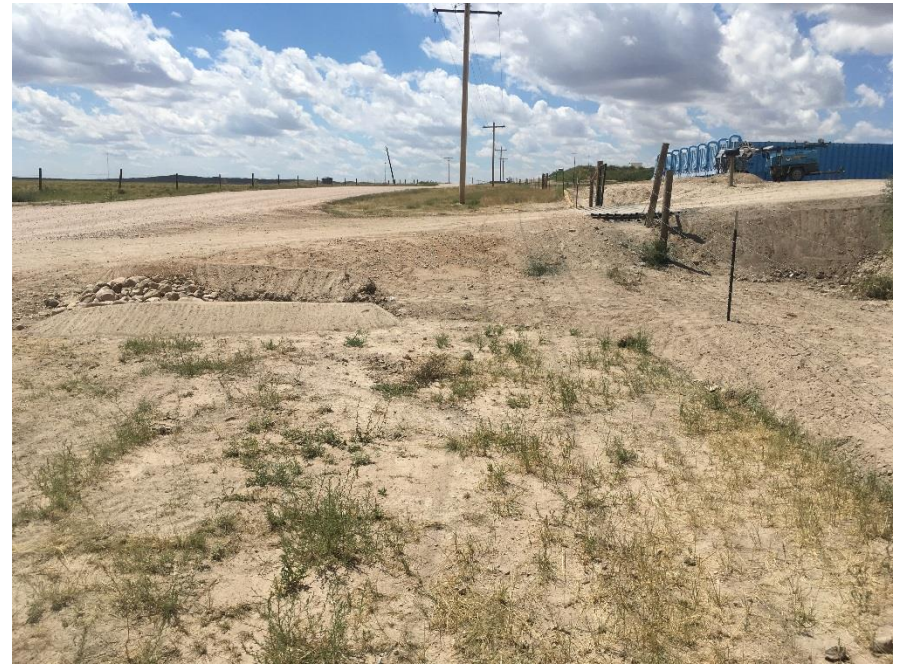
Photo NBL13. The straw wattle was removed and the ditch has been re-cut. The ditch has been extended to the newly installed sediment trap to capture sediment in stormwater runoff from the access road and slope. Weeds have been mowed where accessible, and weeds have been sprayed site-wide. Hydromulch will be reapplied once the weeds have died.
