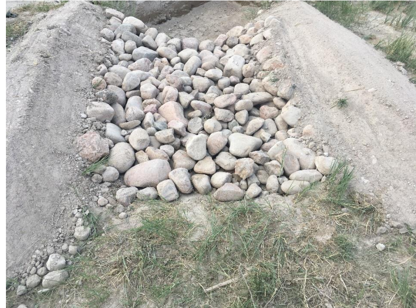
Photo NBL8. The rock outwash was re-installed removing sediment. The sediment trap has been re-installed and enlarged. Sediment traps are used in conjunction with other BMPs as needed to minimize the transportation of sediment in stormwater runoff
