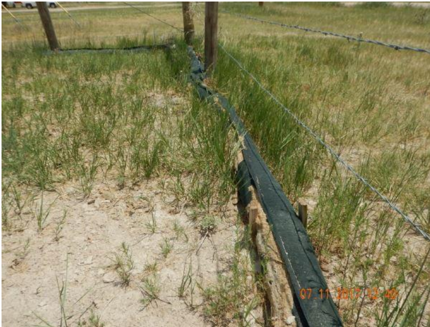
Photo 9. Close up photo taken just beyond the sediment trap at the corner of the fence, illustrating stormwater runoff appears to be washing hydromulch material and sediment off location over the filtrex BMP.
