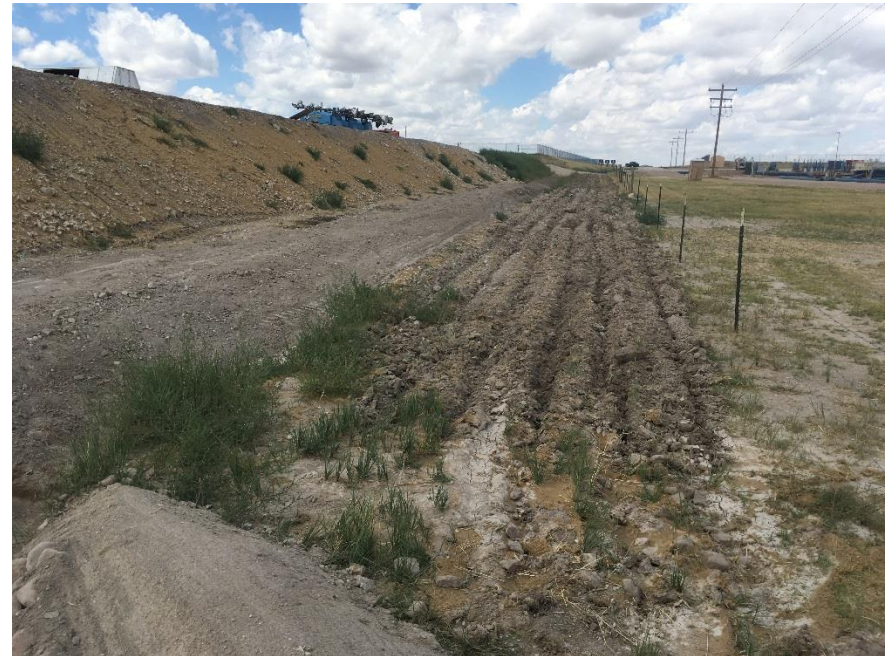
Photo NBL11. The slope has been re-stabilized, the ditch has been re-cut and cleaned out, and surface roughening/ripping was re-installed around the perimeter. Weeds have been mowed where accessible, and weeds have been sprayed site-wide. Hydromulch will be reapplied once the weeds have died.
