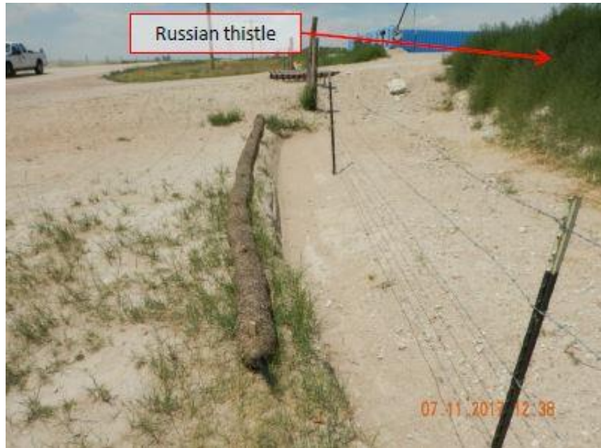
Photo 13. Photo taken from the entrance of the Tombstone pad, facing West. Straw wattle BMP does not appear to be properly installed and therefore not properly functioning.
