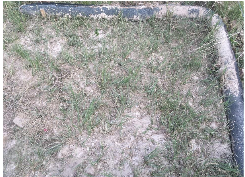
Photo NBL9. Deposited sediment from the area was recovered and the sediment trap prior to the filtrex BMP was enlarged. Refer to photo NBL7
