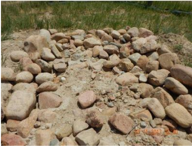
Photo 8. Close up photo taken from the outlet area of the sediment trap illustrating sediment build up which indicate the sediment trap is not built to a sufficient size.
