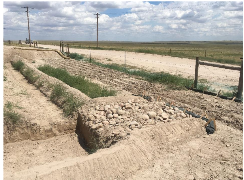
Photo NBL2. Weeds have been mowed where accessible, and weeds have been sprayed site-wide. Once the weeds have died, slopes may be re-sloped and seeded or hydro-mulch may be reapplied for stabilization. The silt fence was not used as a stormwater BMP and has been removed as it was no longer needed for wildlife mitigation.
