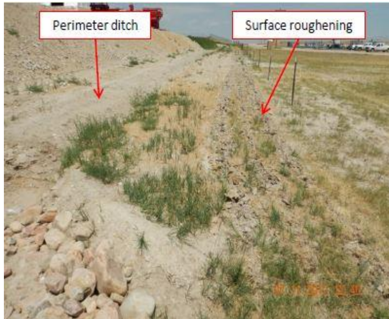
Photo 11. Photo taken from the southeast location of the Tombstone pad, facing North. Perimeter ditch with surface roughening BMP installed along the eastern perimeter. Portions of the fill slope may need additional stabilization as it appears hydromulch does not appear to be consistently observed throughout.
