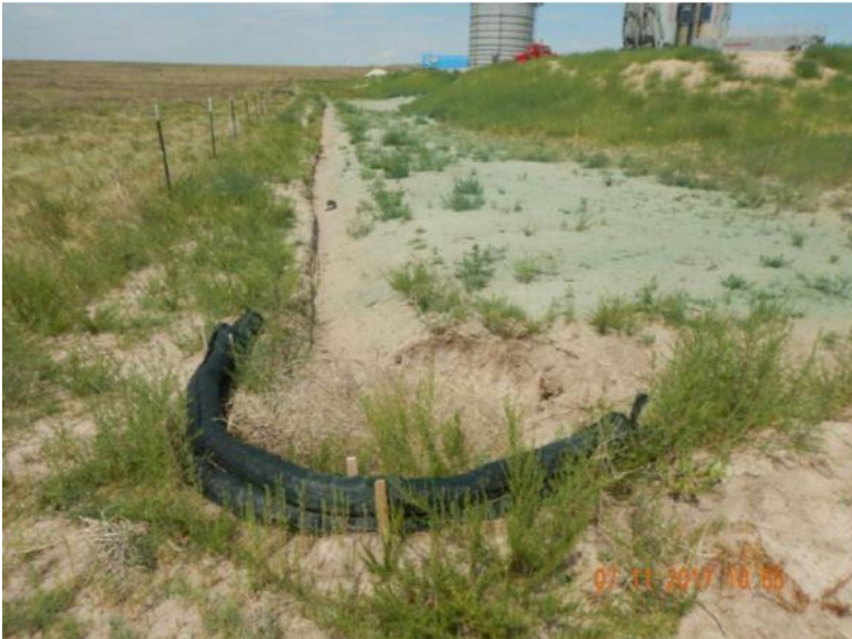
Photo 4. Photo taken from the southeast location, facing West. Sediment trap size was measured at ~6'x6'x2' (width x length x depth= 72ft 3 ) with filtrex at the overflow point of the trap.
