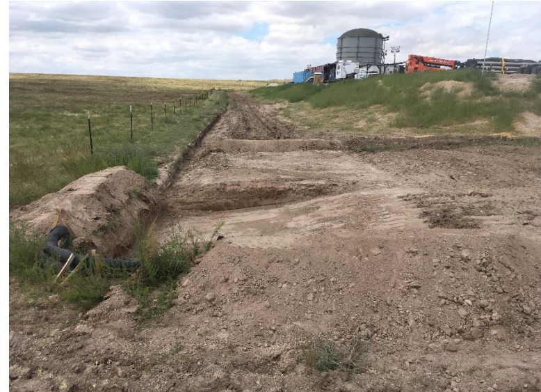
Photo NBL4. The sediment trap was enlarged and the ditches draining to this sediment trap were recut and cleaned out. Sediment traps are used in conjunction with other BMPs as needed to minimize the transportation of sediment in stormwater runoff
