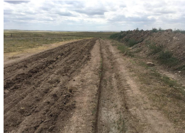
Photo NBL3. Weeds have been mowed where accessible, and weeds have been sprayed site-wide. Ditch was re-cut and cleaned out and perimeter ripping was reinstalled.
