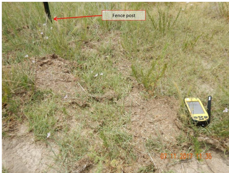
Photo 7. Close up photo taken from the southern perimeter of the location, illustrating stormwater runoff appears to be washing sediment over the ditch and berm BMP off location.
