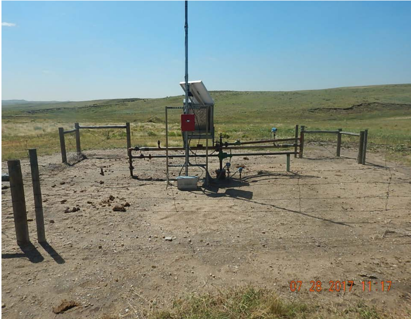
Photo 1: Wellhead, looking S
