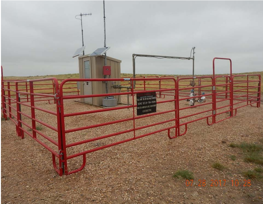
Photo 1: Wellhead, looking NW
