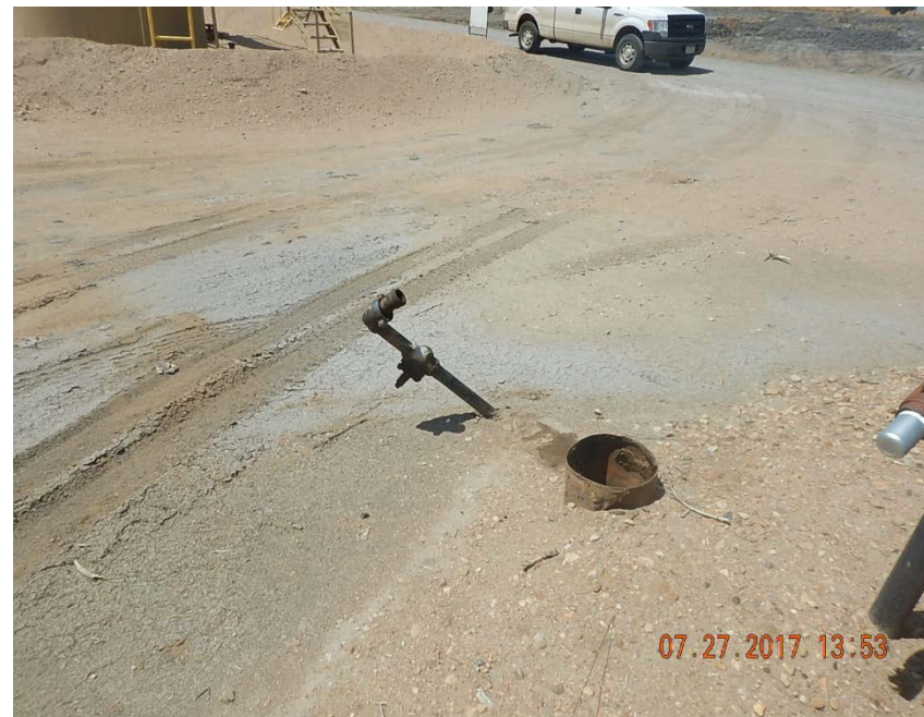
Photo 6: Riser, debris at manifold.
